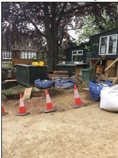
Plate 4 – Materials stored in CEZ and fencing missing adjacent T1.
