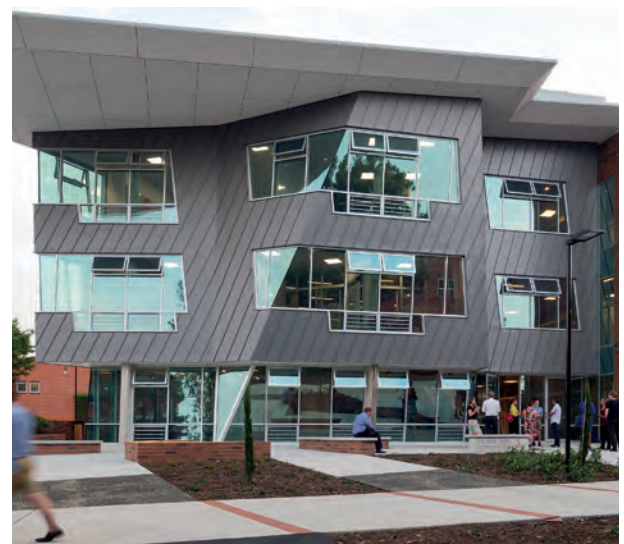
The Snow Centre ACT - Quartz-zinc Standing Seam, Architect: Daryl Jackson Alastair Swain Architects - Installed by Erincole Facade Systems
