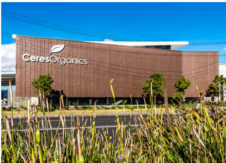
Ceres Building - Auckland - Pigmento Brown Standing Seam, Architect: Williams Architects - Photo: Blair Hastings
