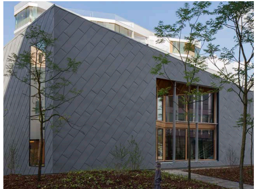
Pastoral House, Boulogne Billancourt France - Designed by Brénac et Gonzales, Installed by CCRT, Bondy - VMZINC Quartz-zinc
