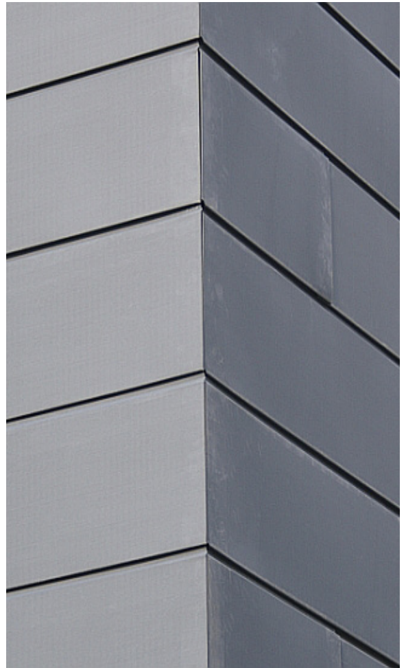
VMZinc Flat Lock Panel Example
