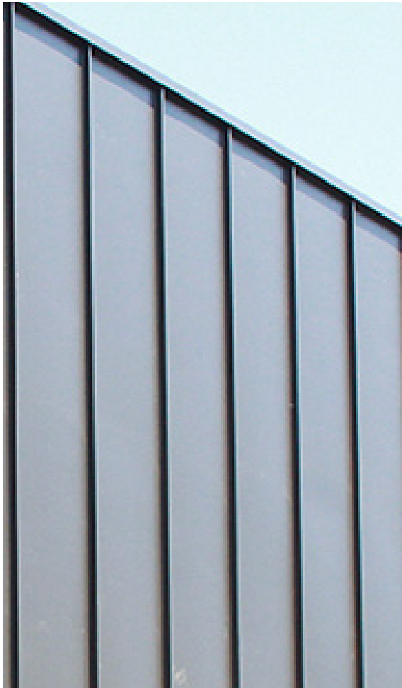
VMZinc Standing Seam Example
