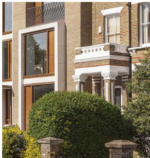
Articulated bays with stone surround, glazing and timber infill panels
