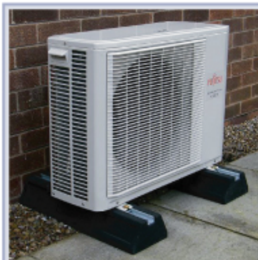
Mounting a condensing unit
