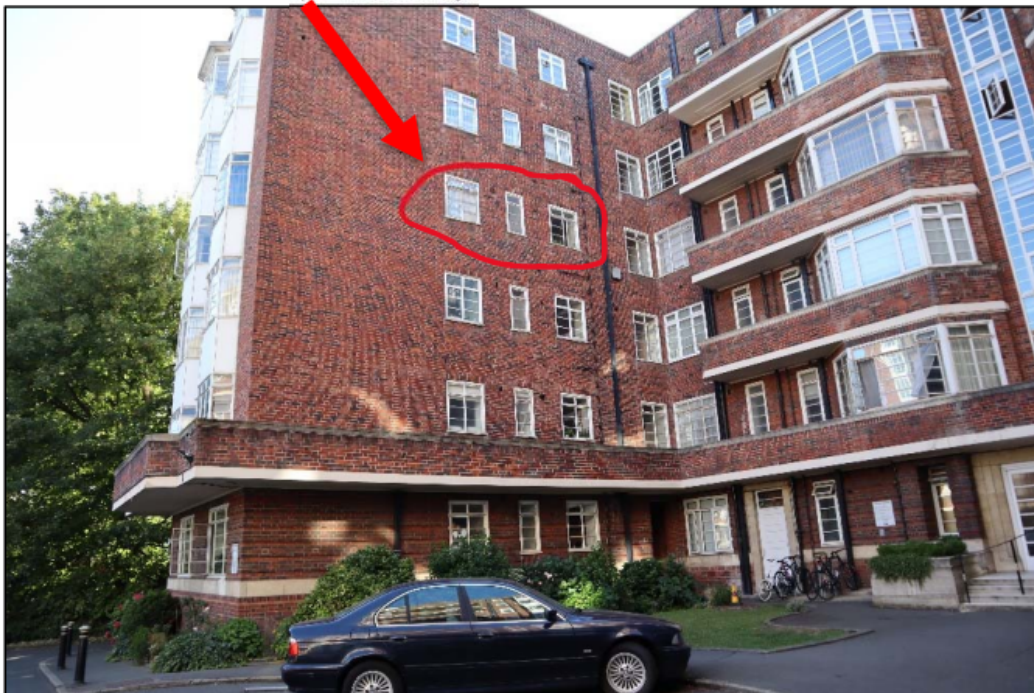
View 2 – north-east elevation showing 3 windows to be replaced
