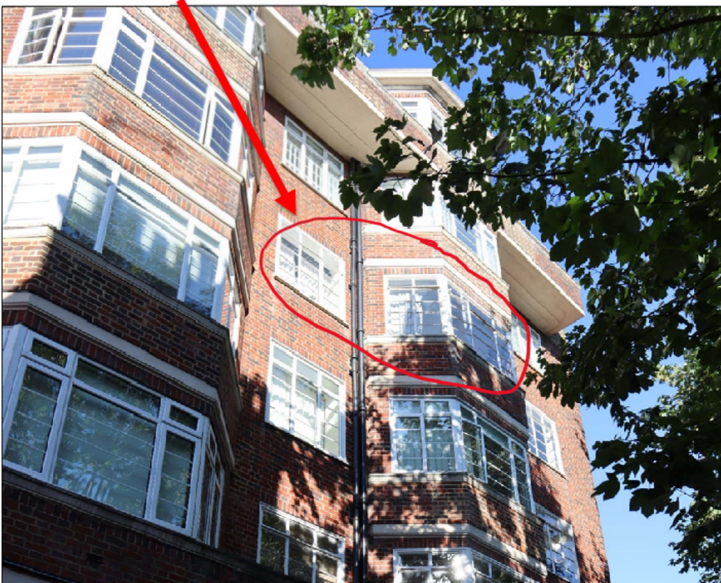
View 1 – south-west elevation showing 4 windows to be replaced
