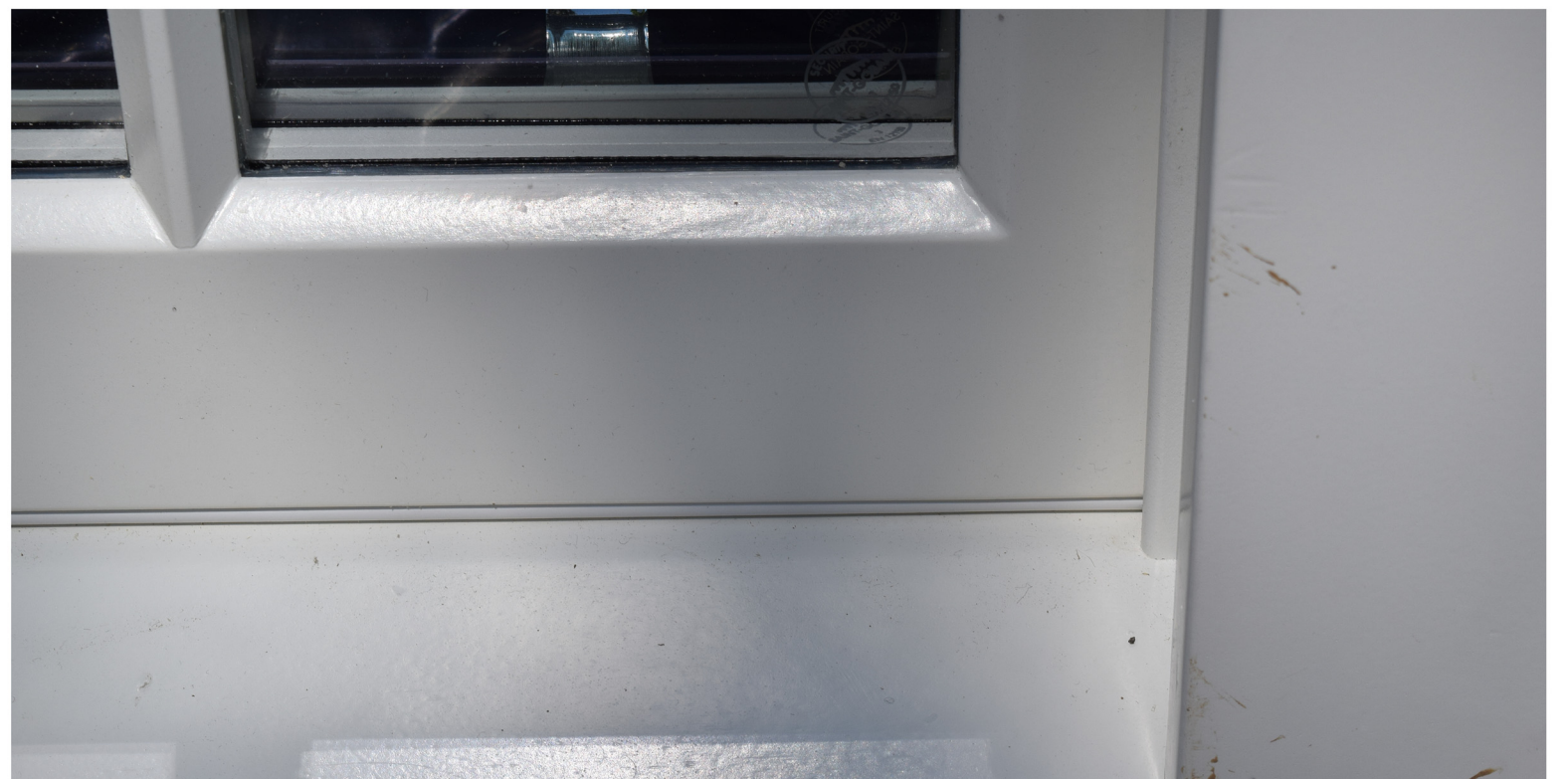
Bottom Sash and Cill
