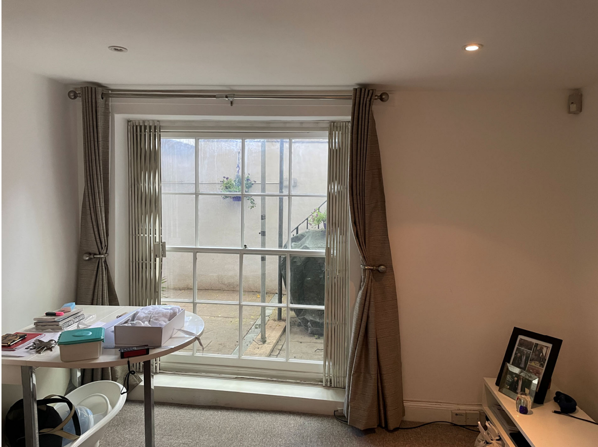
Figure 3 – Internal view of windows within the living room at basement level
