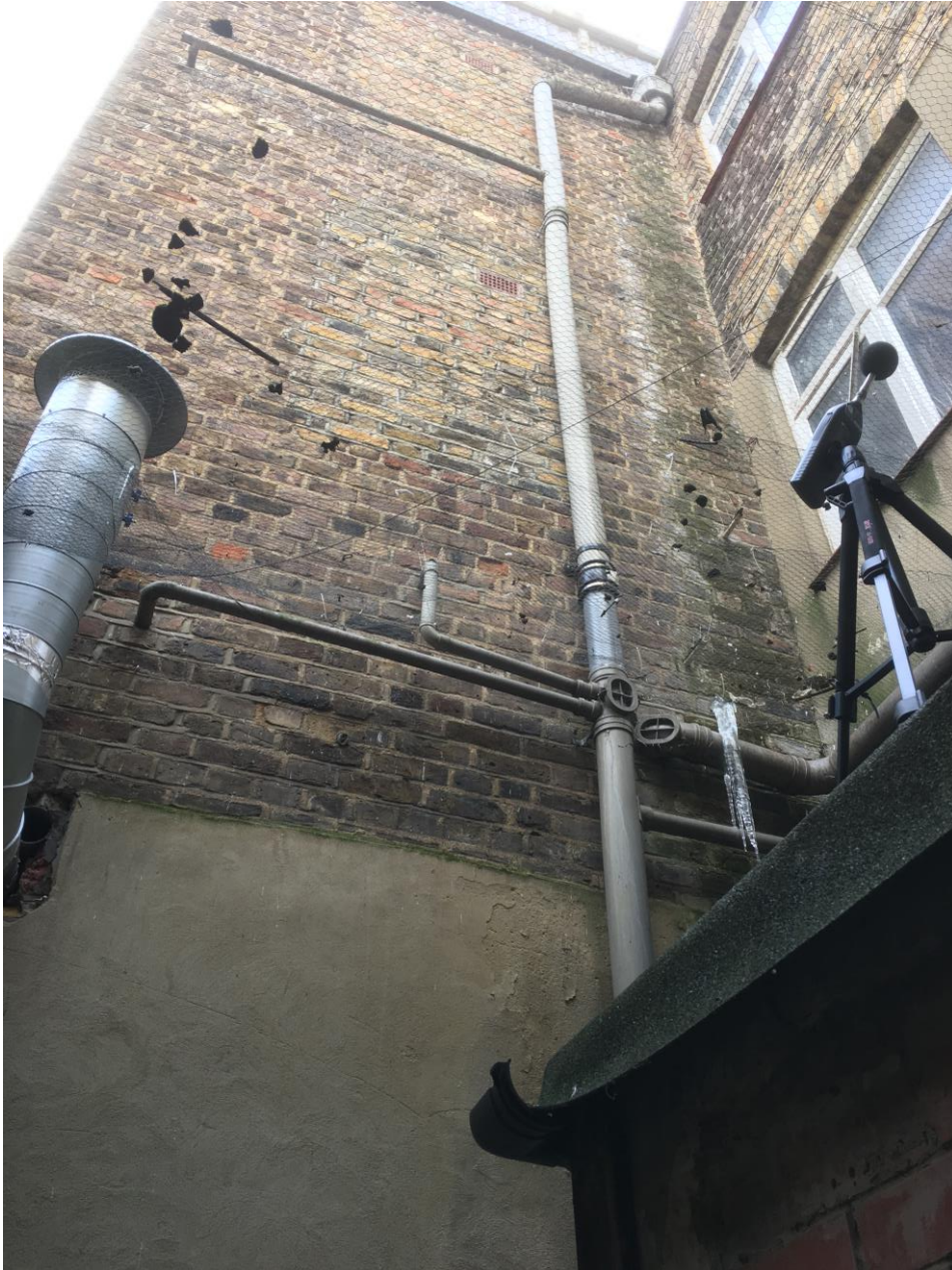
FIGURE A1: EXTRACTION FLUE, RESIDENTIAL WINDOW AND MEASUREMENT LOCATION
