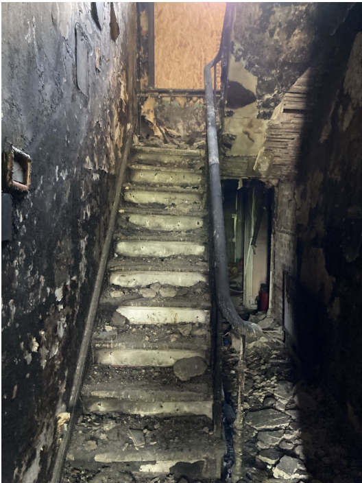
Existing condition internally
