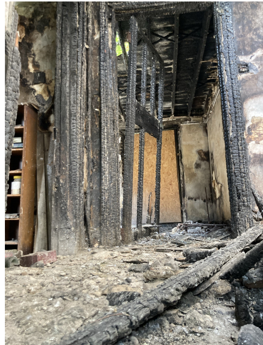
Existing condition internally
