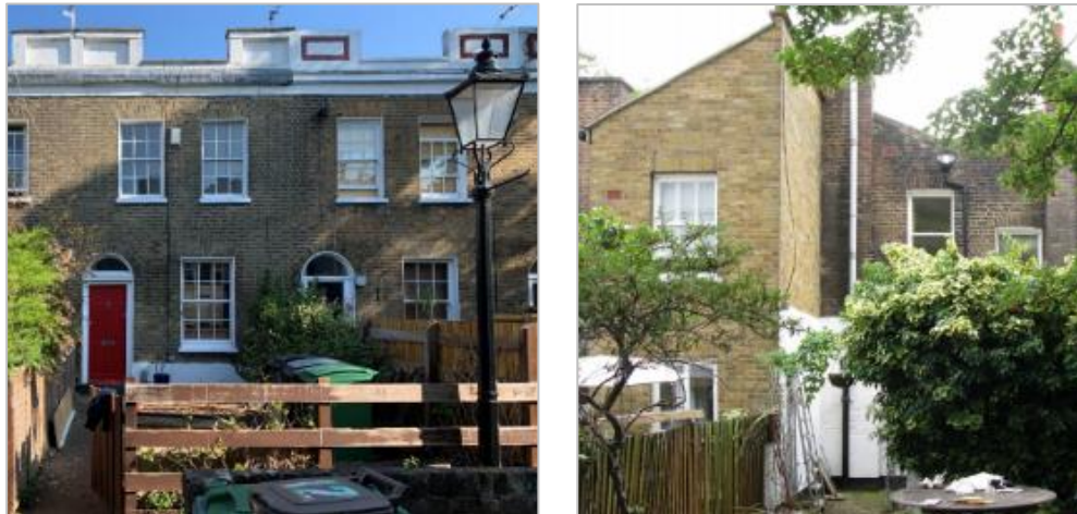
Figure 3: (a) Left - existing principal elevation and (b) right - rear elevation of the appeal site. Note the two-storey mono-pitch extension at no.31 Powlett Place.
