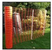
lines), and is to define the access route for foot operatives, to prevent straying into root protection areas other than for hand removal of existing garden room, and to minimise landscape and lawn disturbance. 100mm diameter tops fencing stakes placed at 4m intervals shall be driven at least 0.6m into ground. Plastic barrier material (see left) 1m in height shall be stapled to the stakes.
