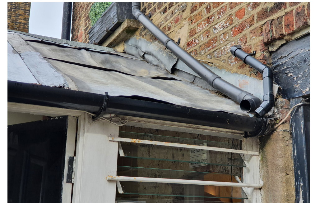
Ad-hoc nature of existing roof to annexe
