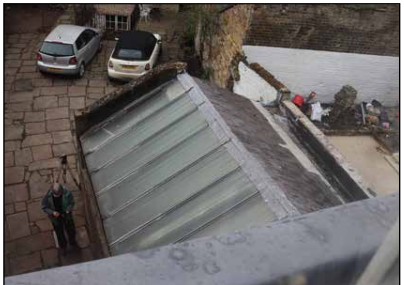
Fig.23. Outbuilding roof with parapet to gable end
