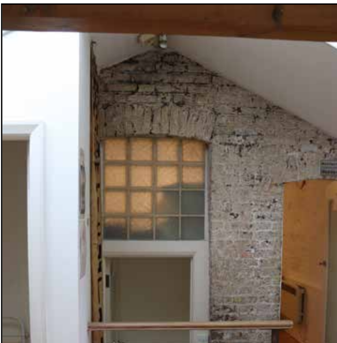
Fig.14 Ground floor rear wall with presumed former doorway (left hand side) and window (right hand side)
