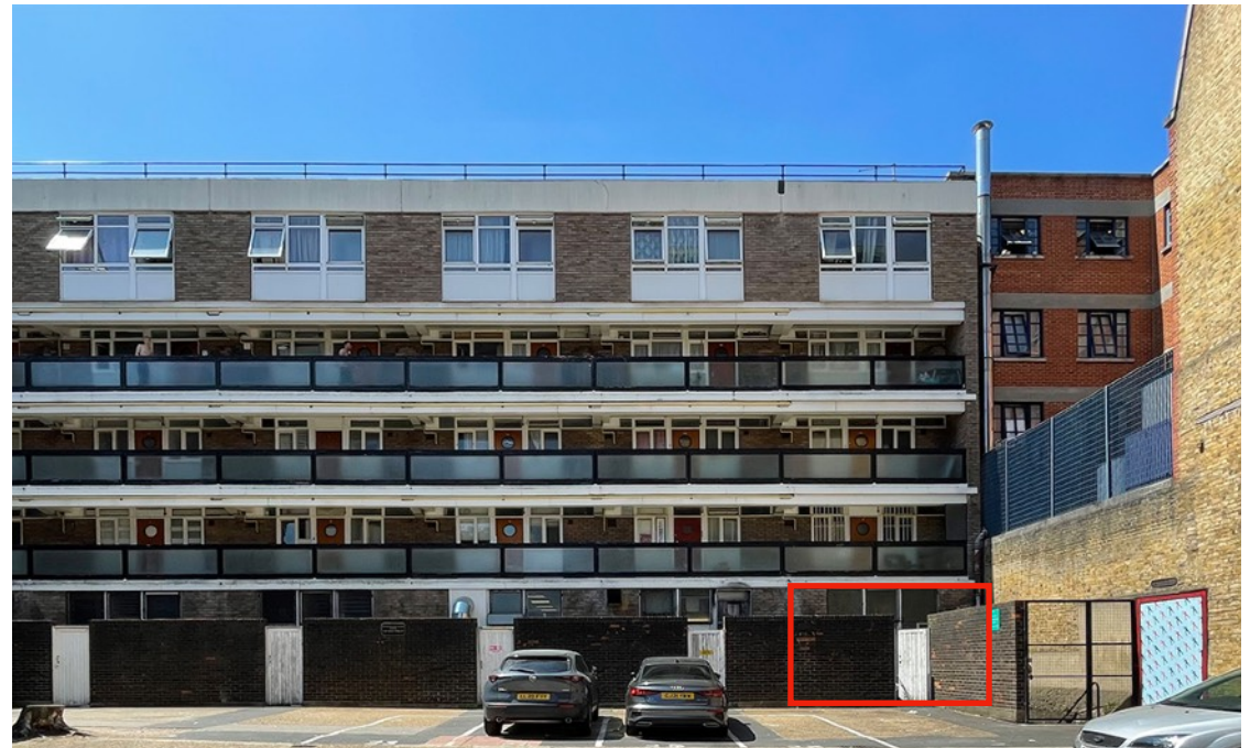
View of the building from rear car park
