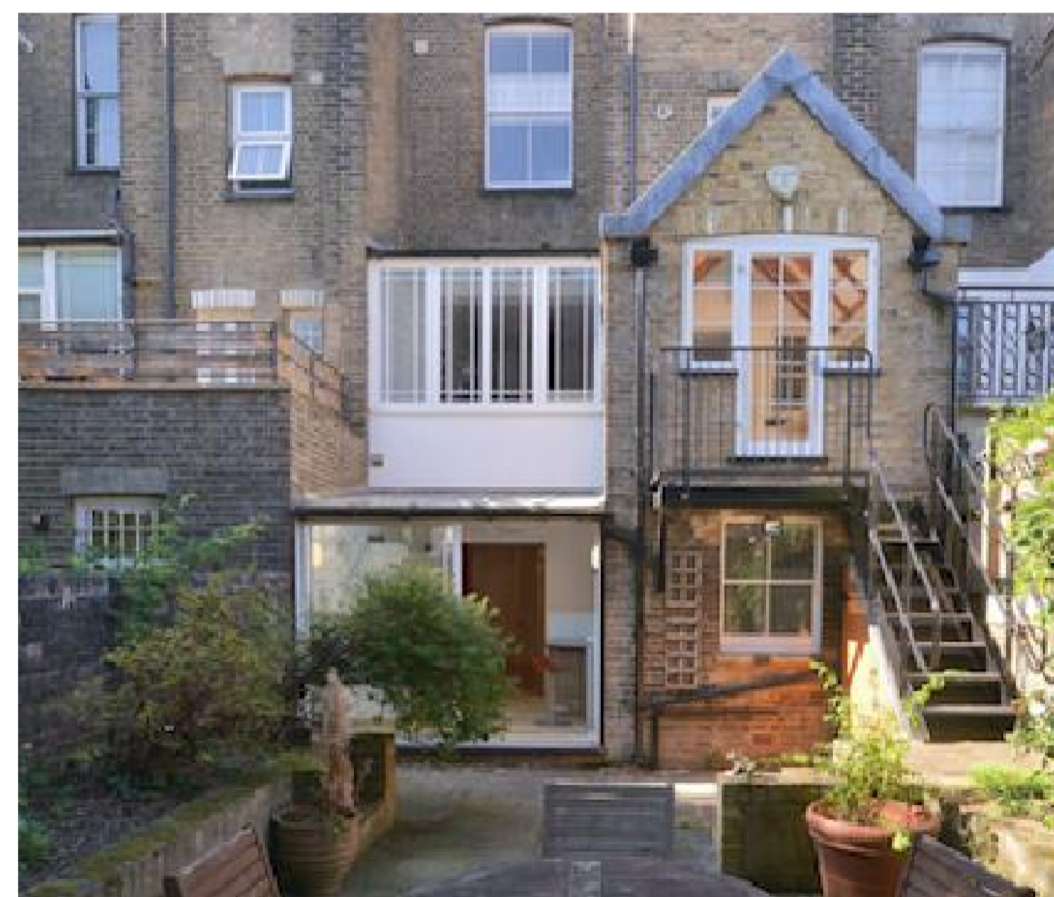
SITE PHOTOGRAPH REAR ELEVATION (LOWER FLOORS)
