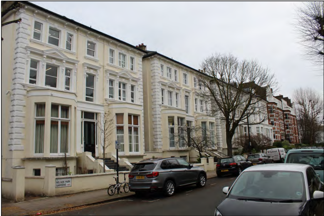
Photo 7: Italianate villas along Belsize Park Gardens, looking east
