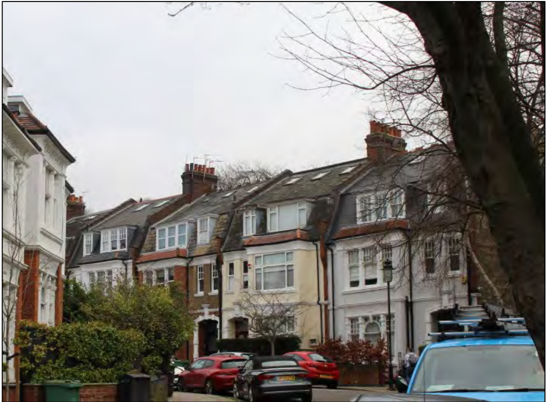
Photo 9: Overview of terrace housing along Howitt Road, looking north-east
