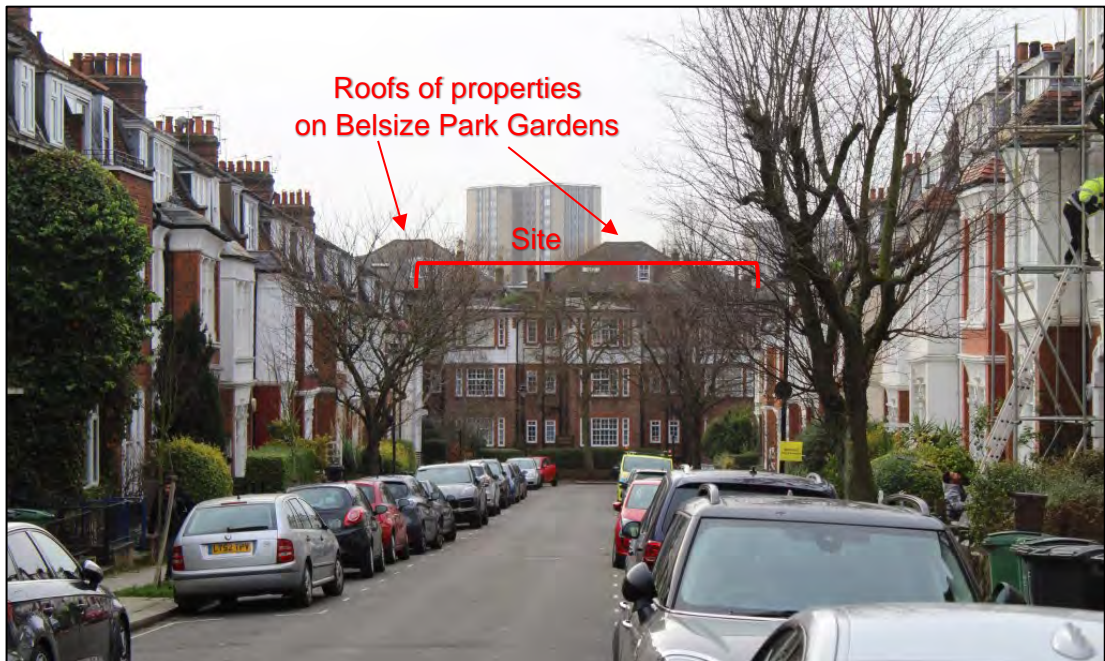
Photo 14: View southwards along Howitt Road, towards the Site
