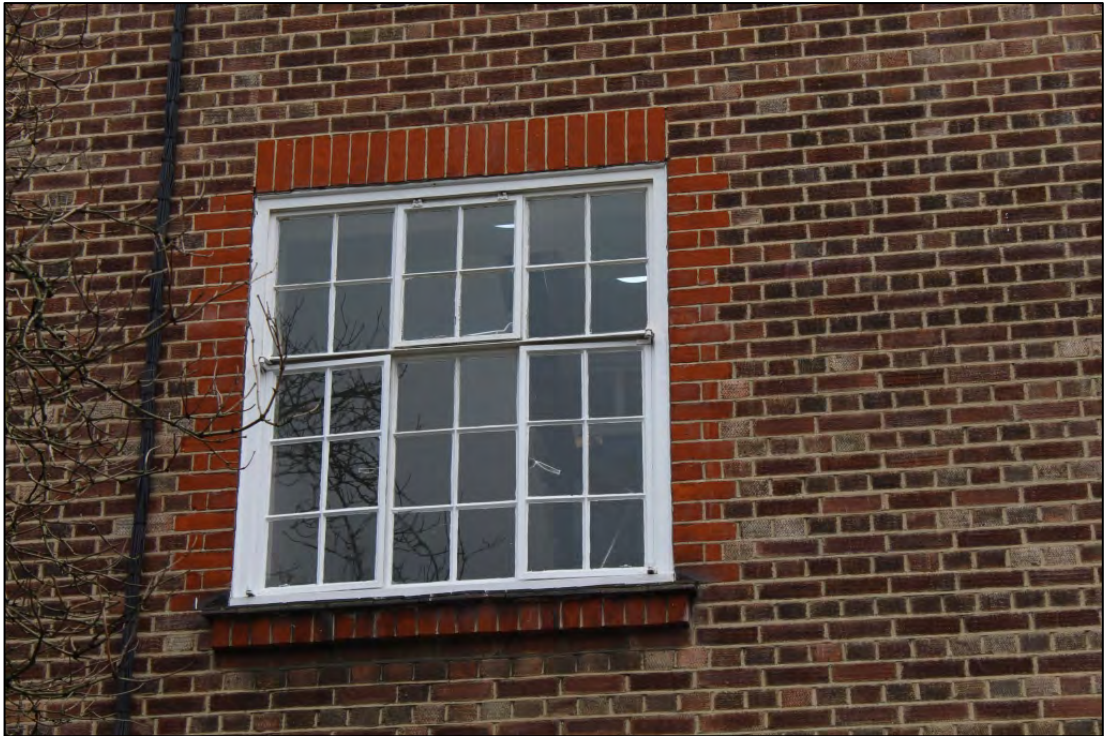
Photo 2: Detail of brickwork to western elevation
