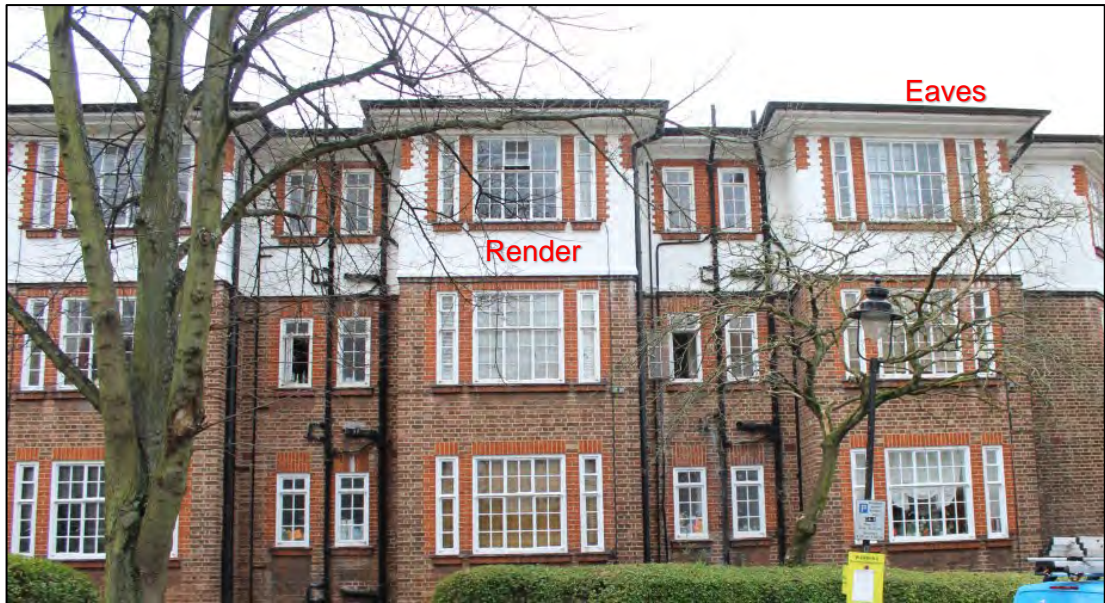
Photo 3: Overview of northern elevation
