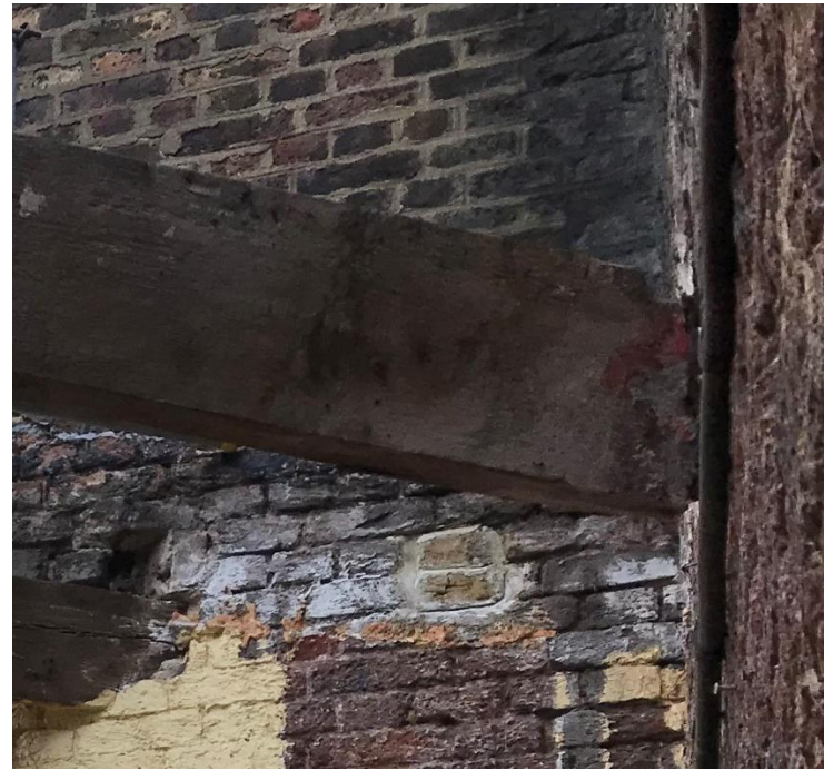
Figure 8 Existing Timber Purlins
