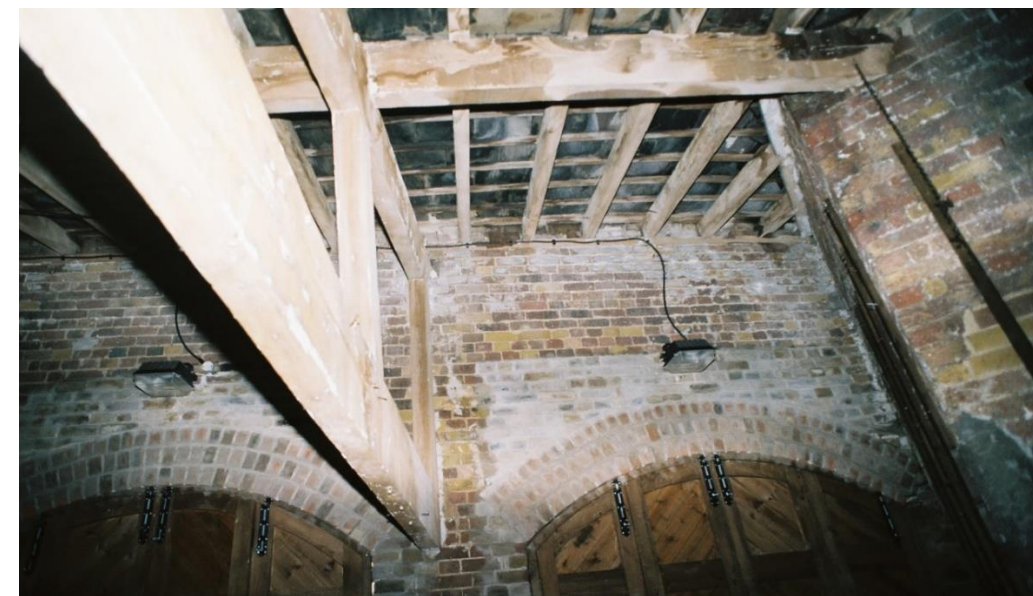
Figure 5 Chalk Farm Road Entrance inside view 1990s
