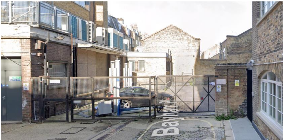
Figure 1. View of hard-landscaped service/parking yard
