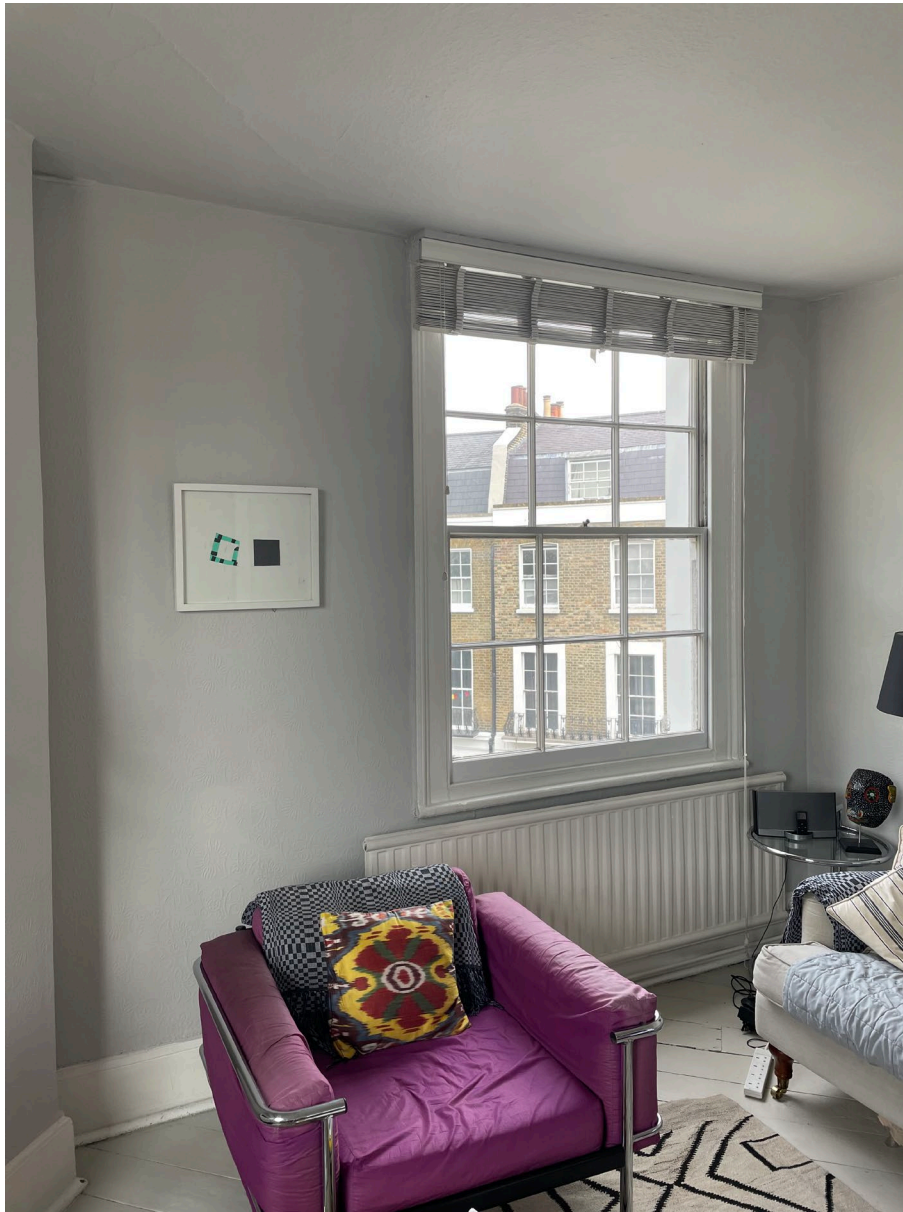
Figure 5: Internal view of right sash window in the living room at second floor
