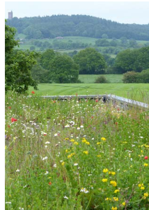
Example of wildflower green roof
