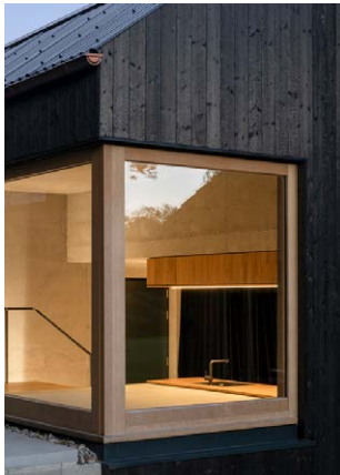
Hardwood timber frame contrasting charred timber facade
