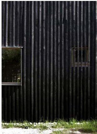
Charred timber vertical louver fins
