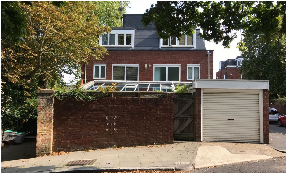
Above: 2 Vane Close as seen from the northwest. Note the corner brick pier in yellow stock which is thought to be part of the front garden walls of the villa that once stood on the site. The conservatory seen above the garden walls is proposed to be demolished and to be replaced by a single storey brick faced extension.
