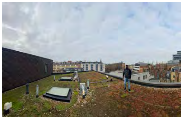
Existing photograph of the current third floor sedum roof
