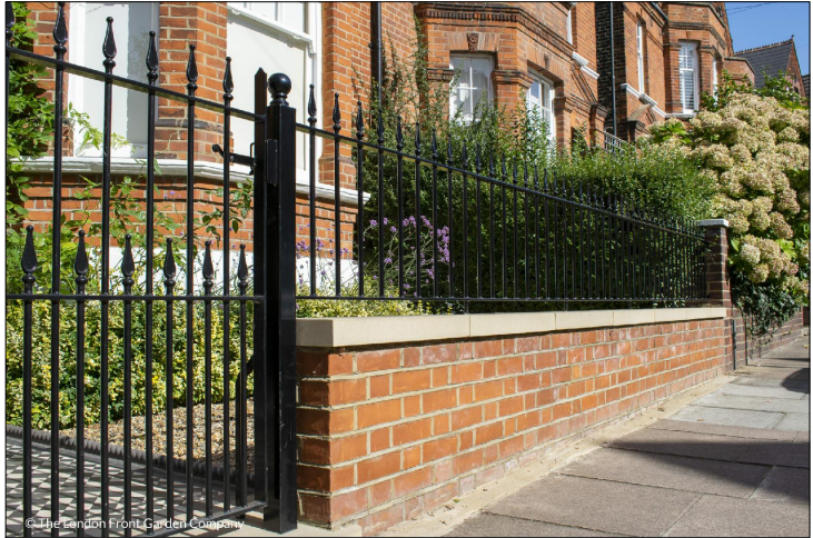
Brick wall buff stone wall coping and railing
