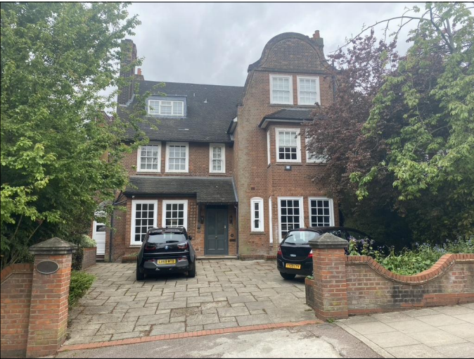
Existing boundary walls and entrance
