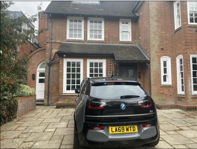
Large area of impermeable hard landscape
