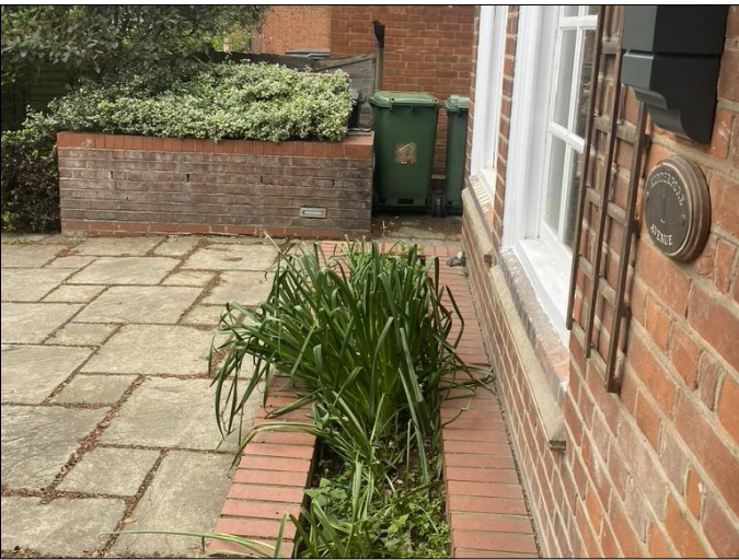
Existing concrete block paving and binstores
