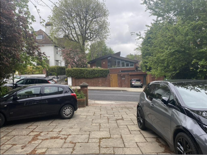
Existing concrete block paving
