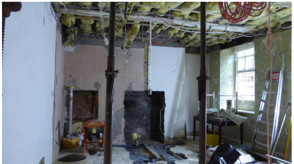
13. The front room following the removal of the ensuite bathroom and corridor wall
