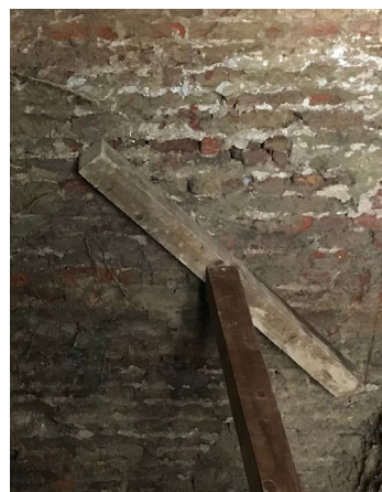
Photo of brick cellar wall propped from inward collapse
