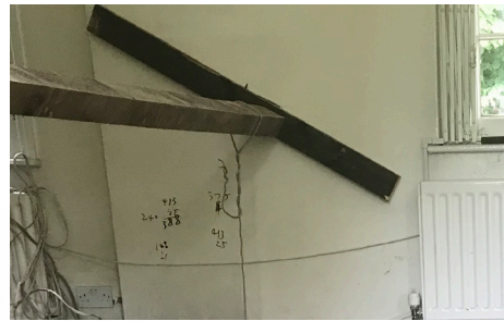
1 Living room walls above cellar propped from inward collapse
