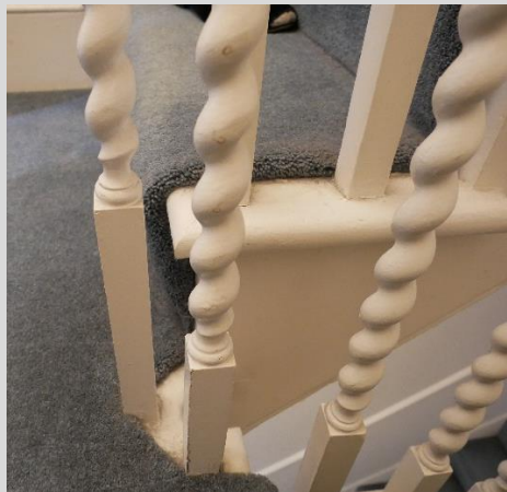
Fig.3 – Existing staircase tread and balusters
