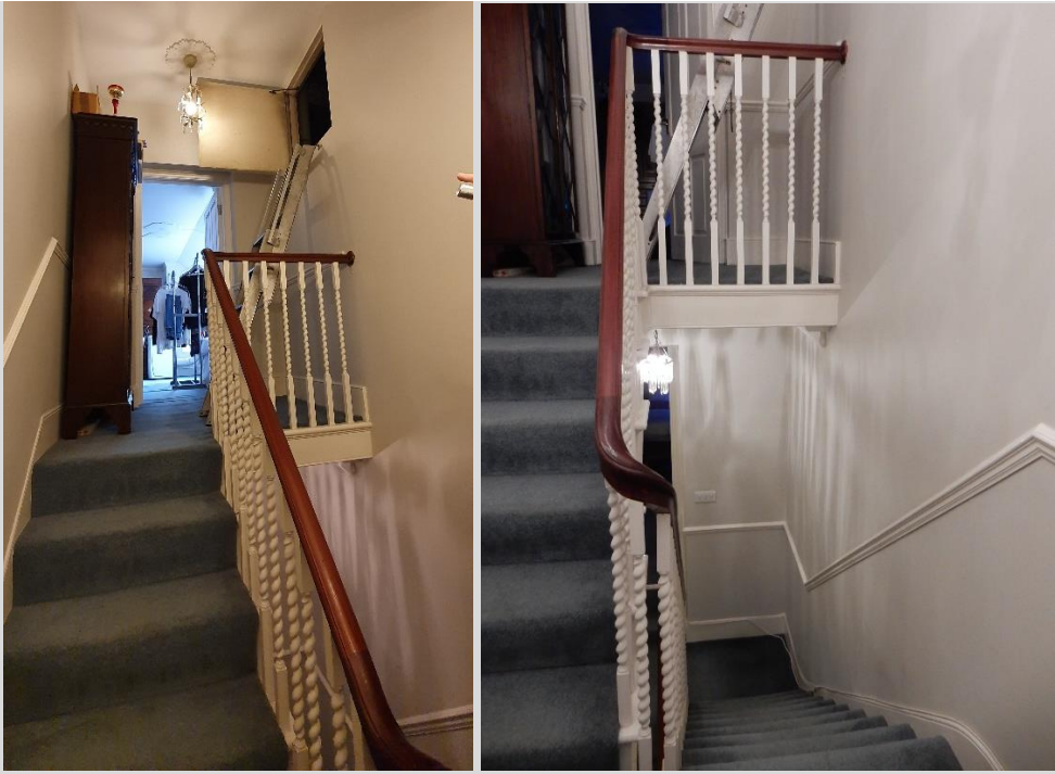
Fig. 1-2 Existing staircase leading to third floor and ladder to loft
