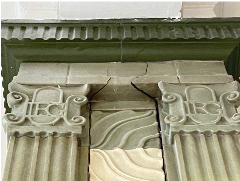
Vertical fractures within the lower cornice.
