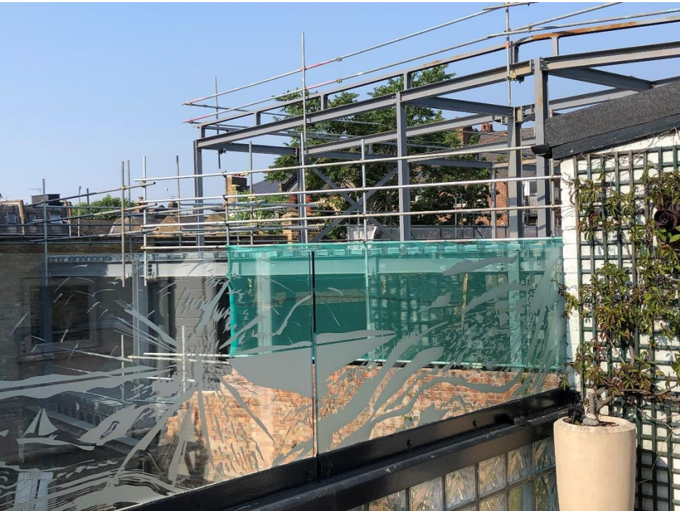
Photo 6: View looking south at application from the roof terrace
