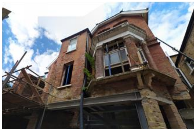
Figure 2: Photo of rear from basement level
