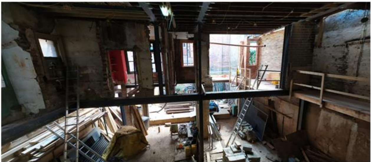
Figure 1. View of excavated basement which extends to rear boundary
