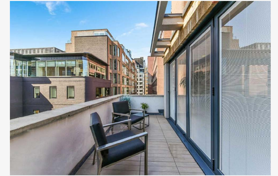
Existing roof terrace
