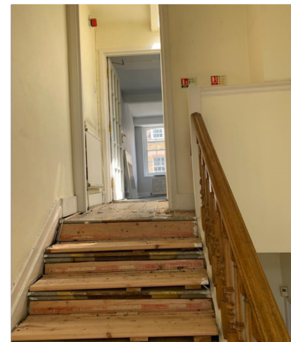
Historic levelling of the original stairs
