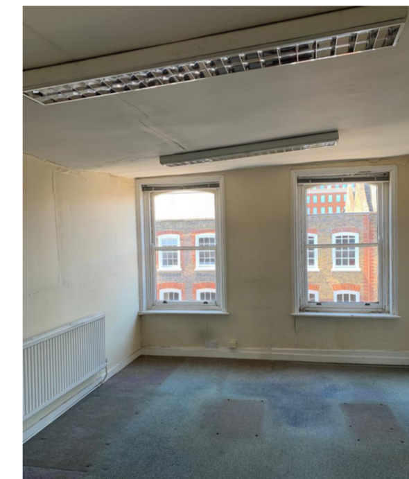
Fourth Floor Office Space
