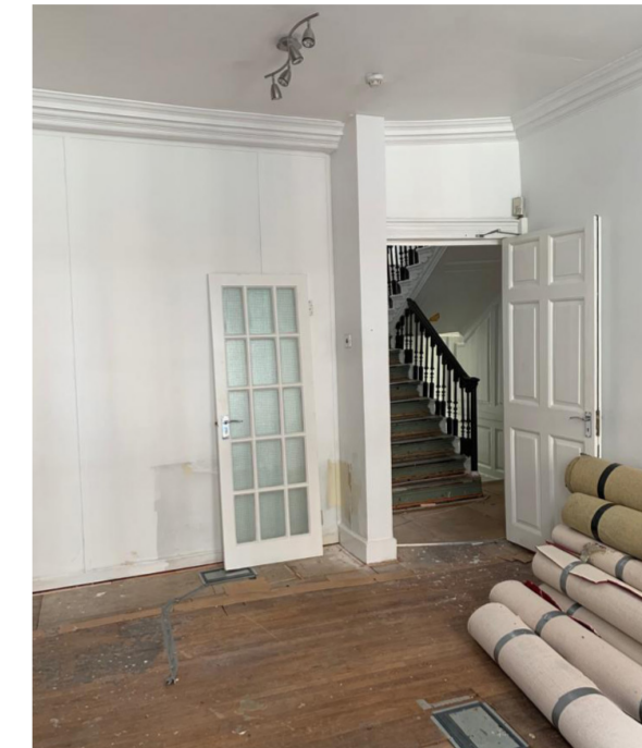
Existing first floor office space, requiring extensive refurbishment
