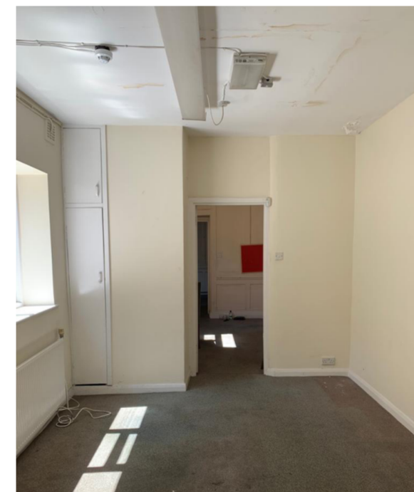
Surface mounted wiring and fluorescent lighting, non original windows
