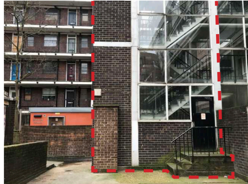
Existing Devonshire Court stair core and position of new lift (in red)
