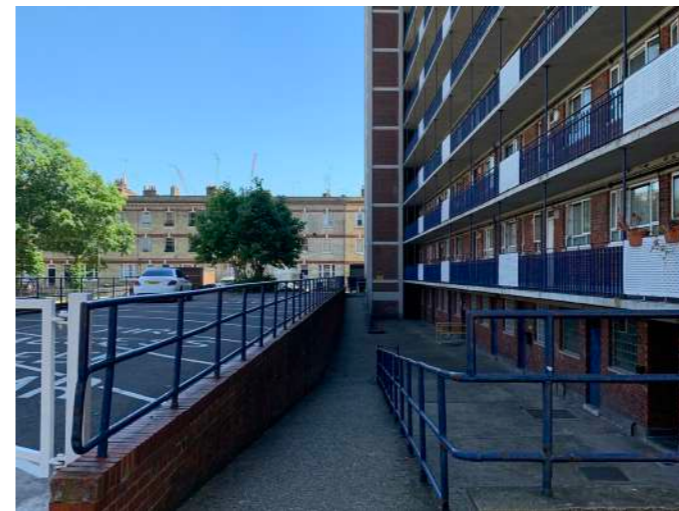
6. Blemundsby Block - Ramp to underbuilds.
