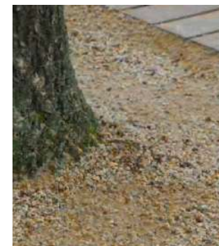
P7. SuperCEDEC Tree pit gravel, colour gold, laid to a compacted depth of 50mm.
