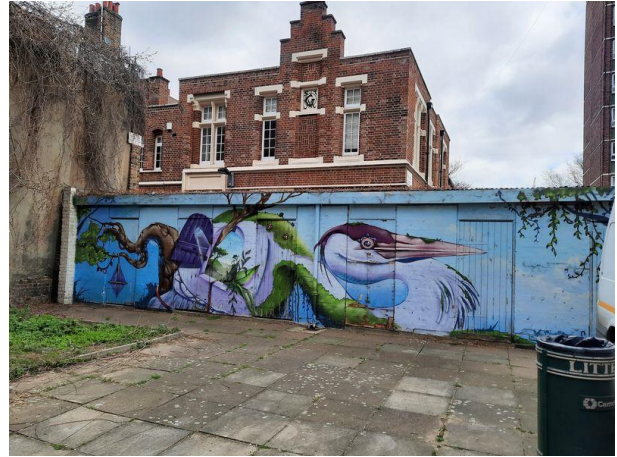
Plate 9.2: Building with Fencing and Hardstanding
