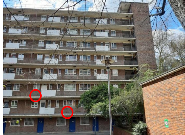
Plate 4.20: Extent of Airbricks (Building B7, Eastern Elevation)
