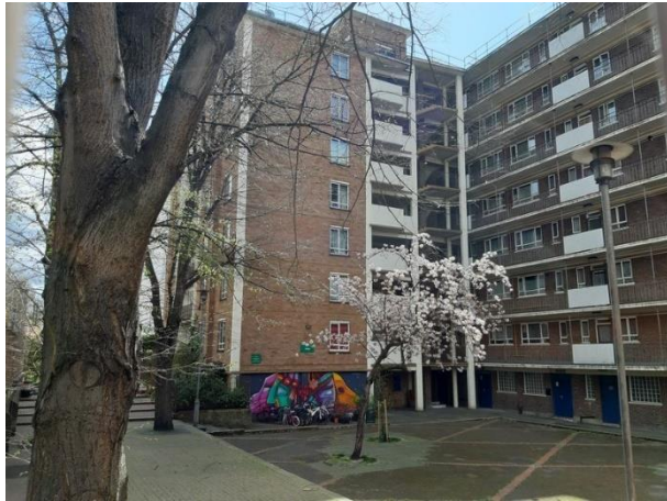
Plate 4.15: Building B7 - Falcon (North-Eastern Elevation)
