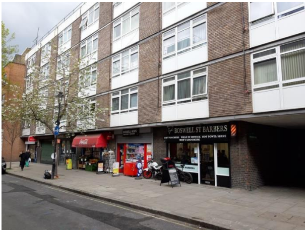
Plate 4.21: Building B8- Devonshire Court (Southern Elevation)
