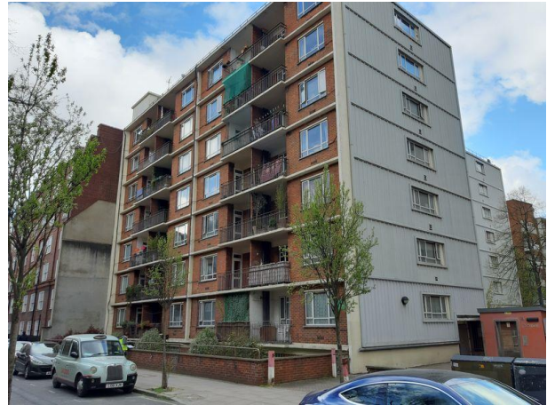
Plate 4.12: Building B6 – Richbell (Southern Elevation)
