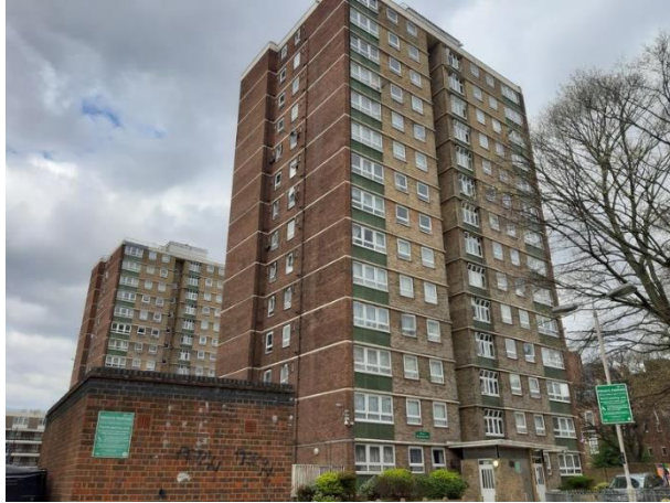
Plate 4.3: Extent of Painted Fascia Board and Roof Storage Building (Eastern Elevation)
