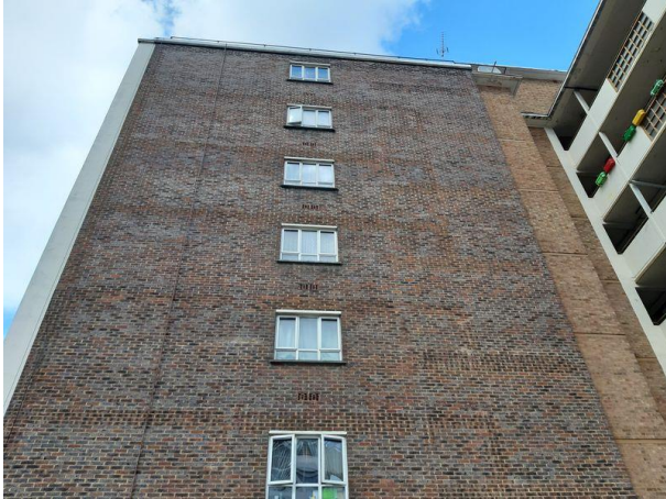
Plate 4.19: Extent of Airbricks (Building B7, Southern Elevation)
