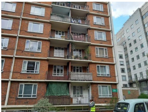
Plate 4.13: Extent of Airbricks (Building B6 – Richbell, Western Elevation)
