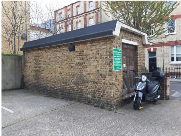
Plate 4.27: Storage Building (Western Elevation)
