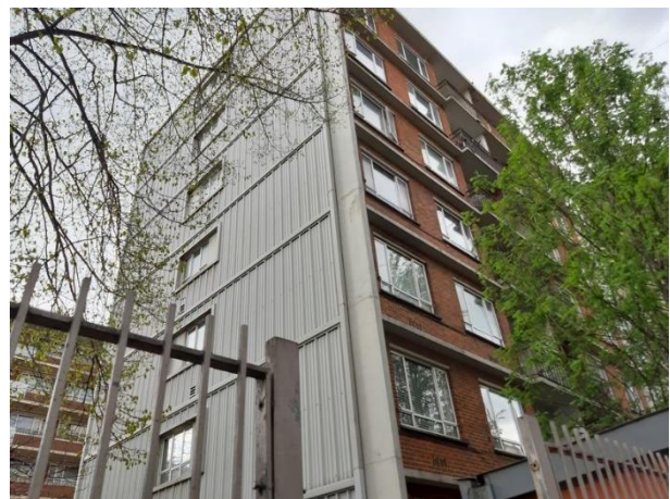
Plate 4.14: Air Vents on Prefabricated Metal Wall (Building B5 – Springwater, Southern Elevation)
