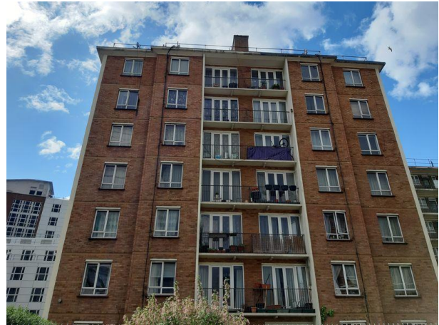
Plate 4.16: Building B7- Falcon (South-Eastern Elevation)
