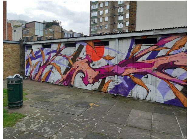
Plate 4.32: Storage Shed (Eastern Elevation)
