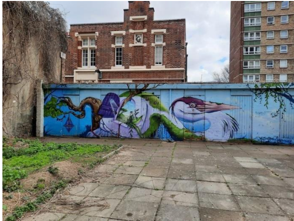
Plate 4.31: Storage Shed (Western Elevation)
