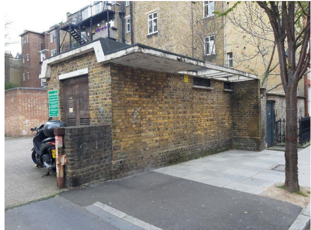
Plate 4.28: Storage Building (Eastern Elevation)
