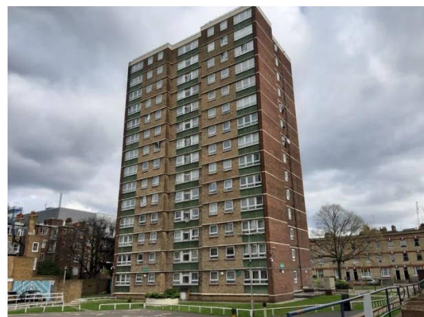
Plate 4.2: Building B2 - Chancellors' Court (Western Elevation)
