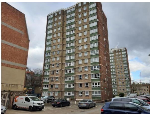
Plate 4.1: Building B1 - Babington Court (Western Elevation)
