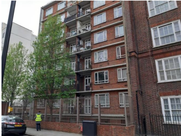
Plate 4.11: Building B5 – Springwater (Eastern Elevation)
