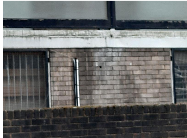
Plate 4.24: Open-ended Pipework (Eastern Elevation)
