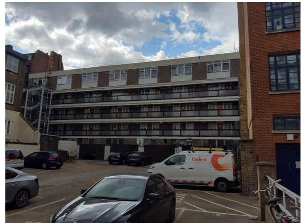
Plate 4.22: Building B8 – Devonshire Court (Eastern Elevation)
