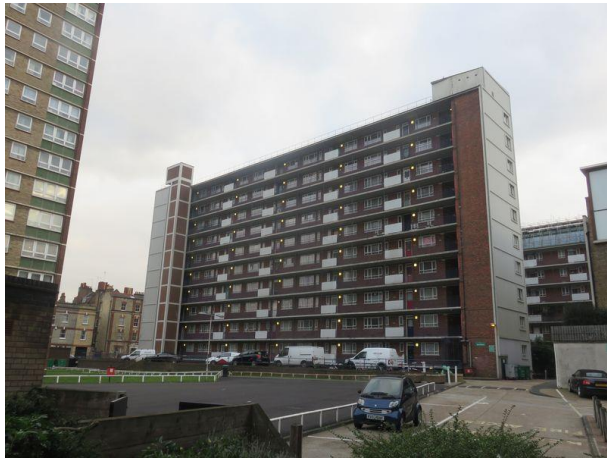
Plate 4.7: Building B3 – Blemundsbury (Northern Elevation)
