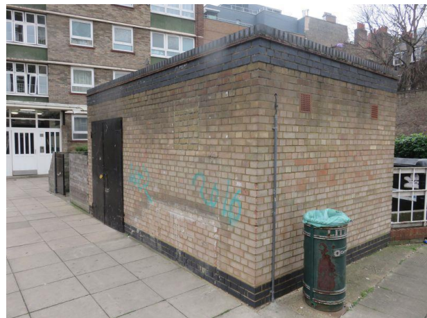
Plate 4.30: Storage Building (Southern Elevation)
