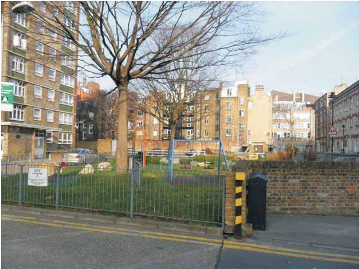
Plate 5: View from Orde Hall Street showing Chancellor's Court and Play Area
