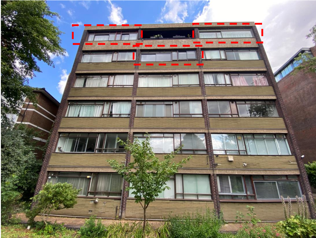
Rear elevation (center part)
