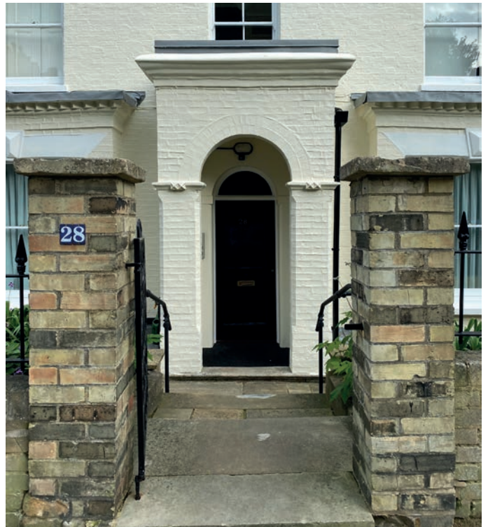
Existing front steps with handrails on each side. The treads to the steps are heavily worn, the coping stones and bottom pilers are in poor condition.
