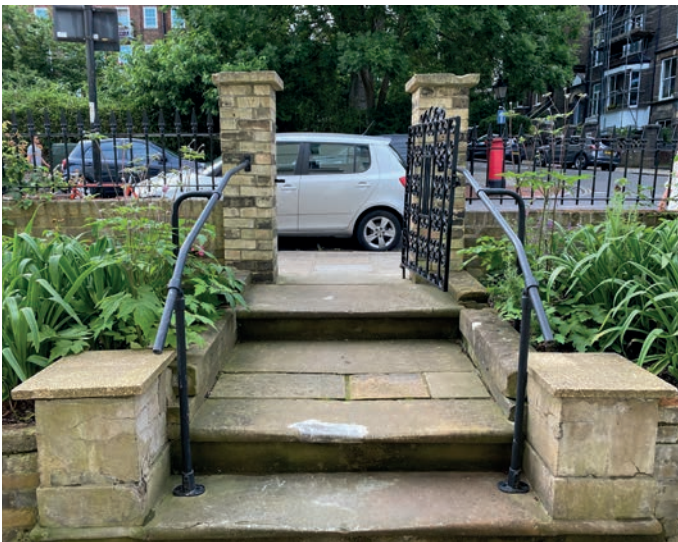
Existing front entrance piers with flat coping stones.
