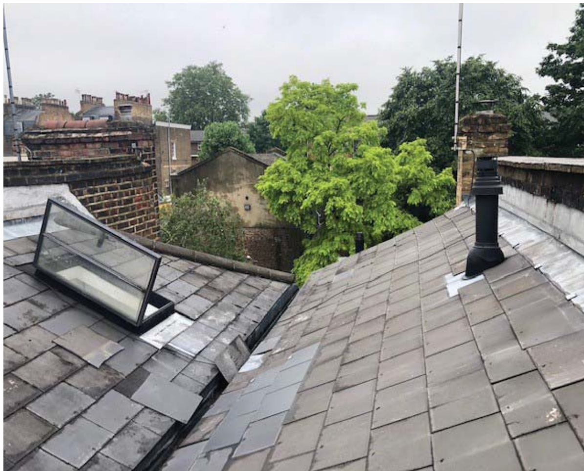
9. View of rear roof looking west. Noted is the southern half of roof is hipped towards the rear (left hand side in this photograph) and the northern half of the roof has a valley shape (right hand side in this photograph).
