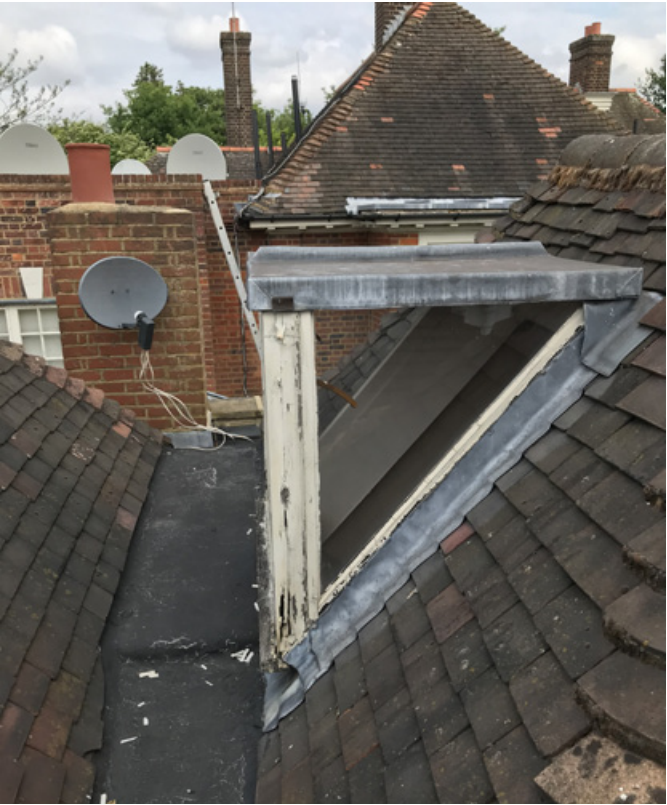
Hidden dormer in poor condition; to be replaced
