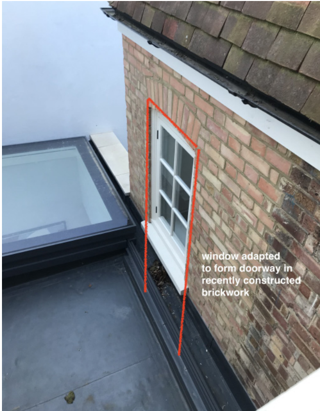
External view of window to be adapted to form doorway
