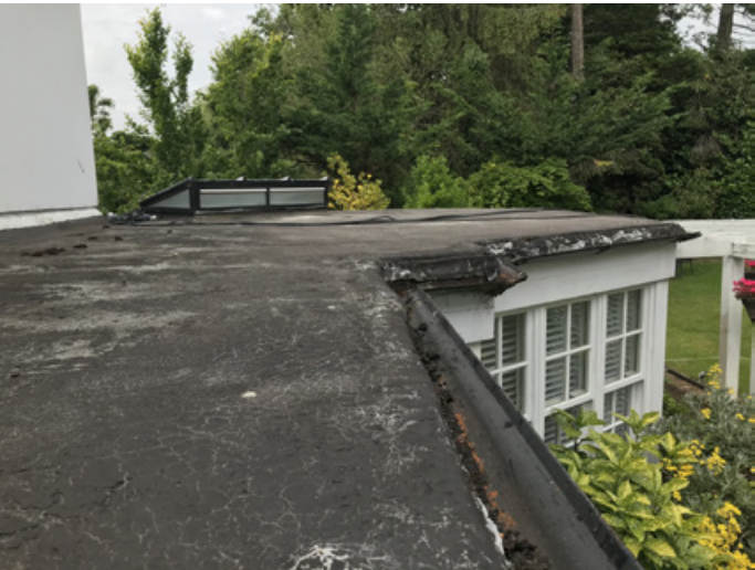
Asphalt roof to kitchen extension in poor condition. To be replaced with new lead roof. Note also lantern ligh - to be removed
