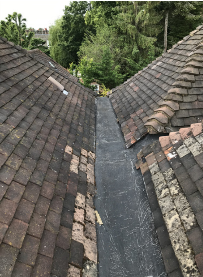
Hidden dormer in poor condition; to be replaced
