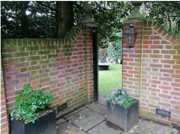
Existing walled area to be taken down. Brickwork is laid in cement mortar and is of recent origin.
