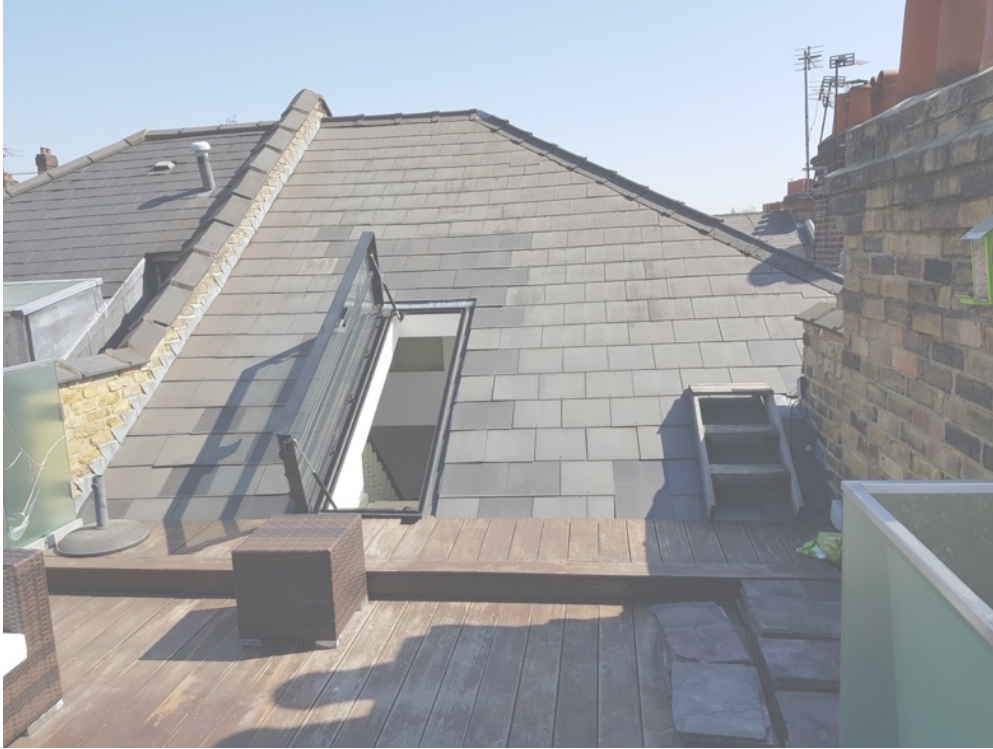
Photo 7: View of Existing Roof Terrace (taken 19 th April 2021)
