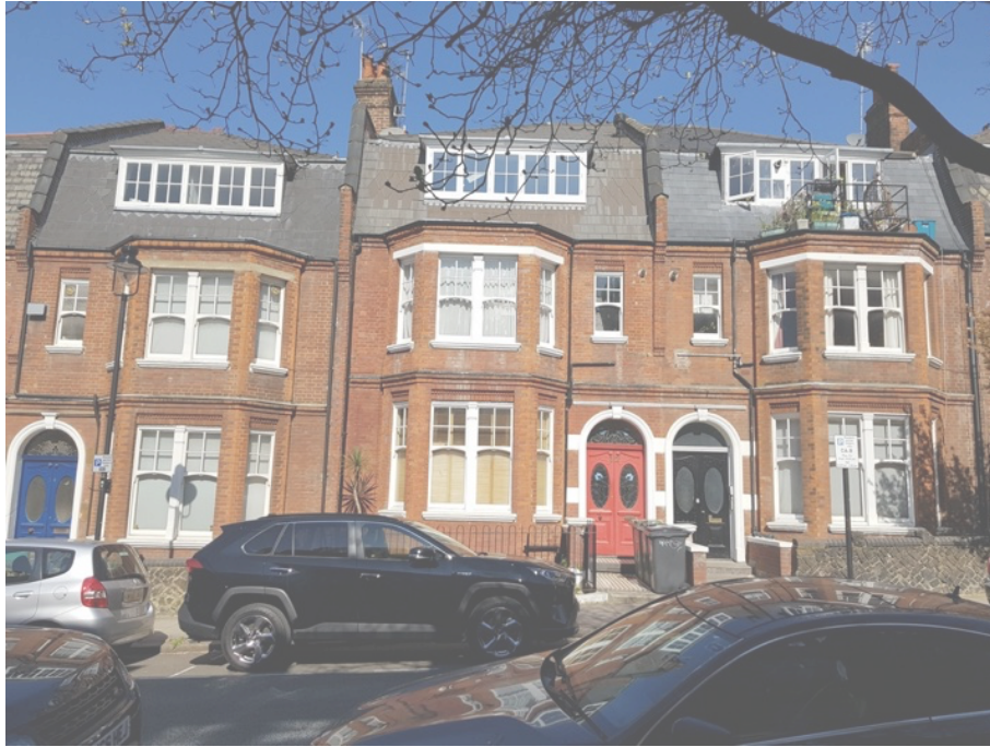
Photo 1: 32 Glenloch Road Street View (taken 19 th April 2021)
