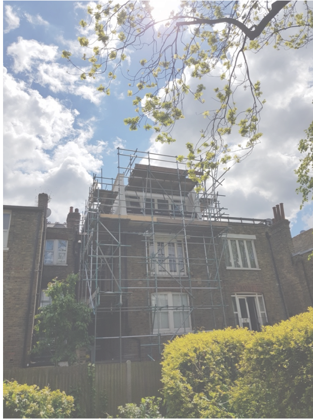
Image: 48 Genloch Road (Roof dormer with doors)
