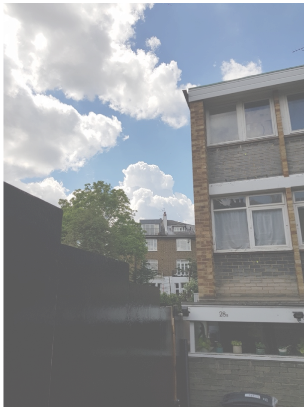
Image: View South West from Glenilla Road (Roof dormer with doors)
