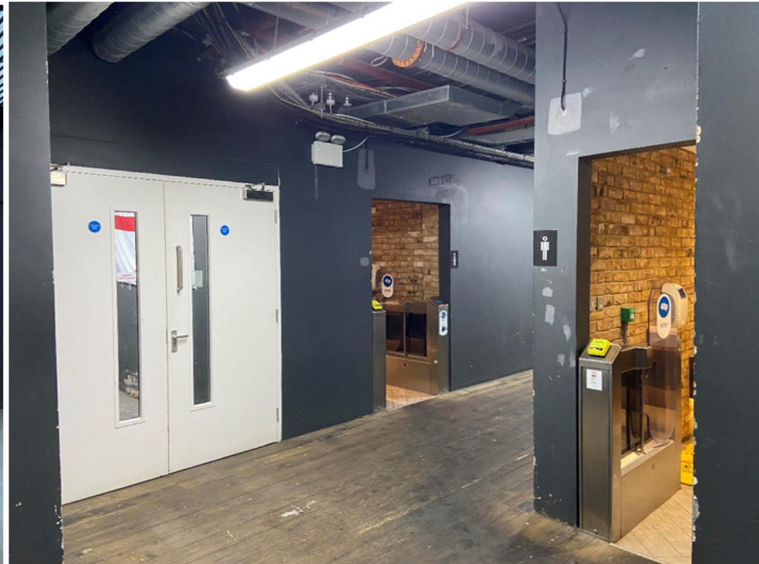
Lift arrival view at basement level
