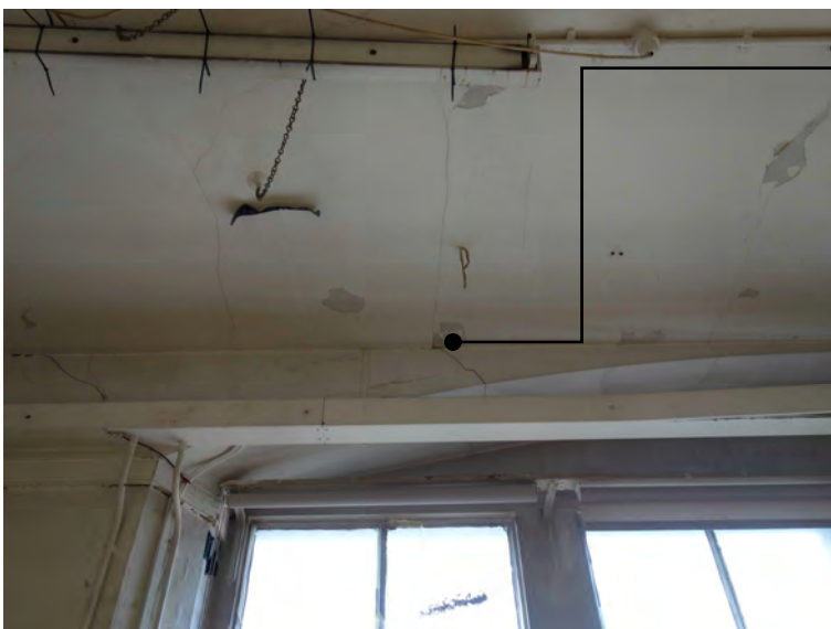
3.6 Cracking to the plaster beneath the steel joists extends into the window arch.
