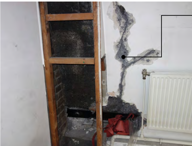
5.19 An area of clinker concrete has been removed exposing the steelwork within.
