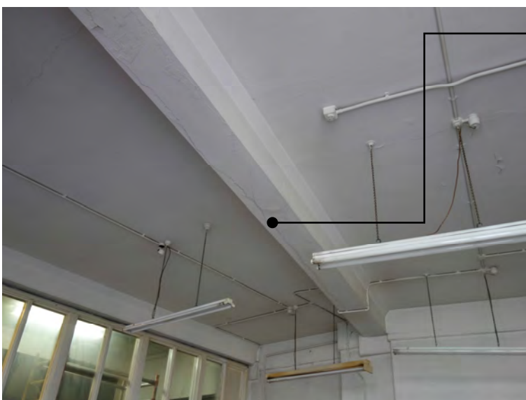
1.2 Cracking can be seen along the length of the beam.
