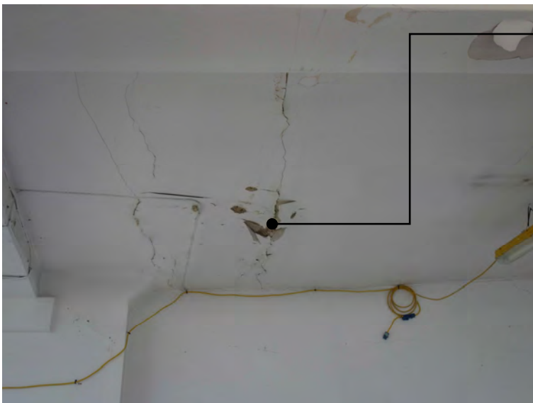
5.11 A large crack is evident beneath an assumed joist location.
