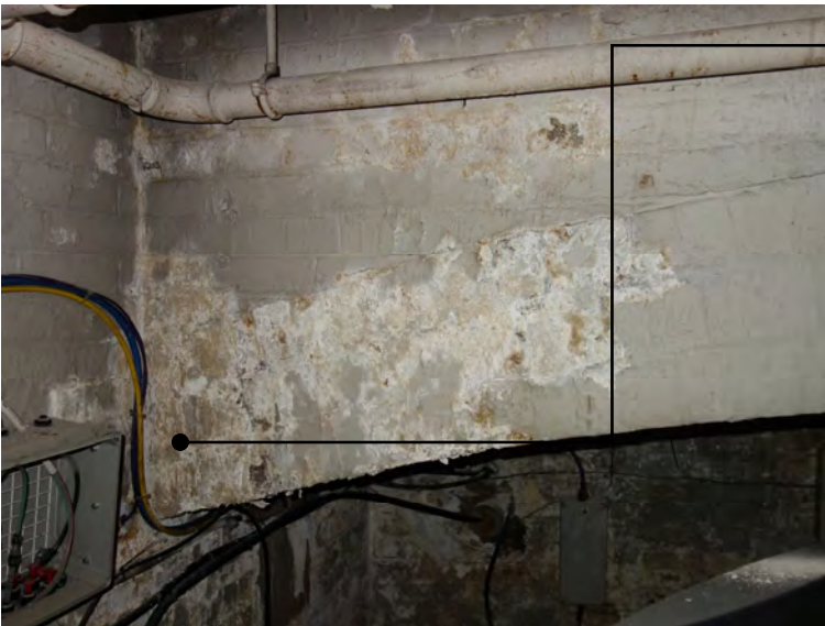
B.9 Water ingress and significant damp found in pavement vault.
