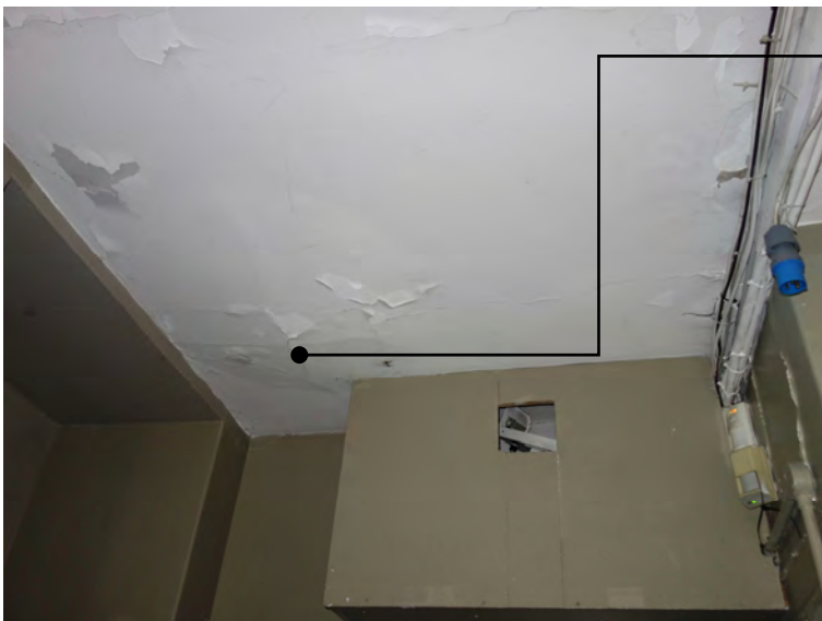
G.3 Water ingress noticeable at high level.
