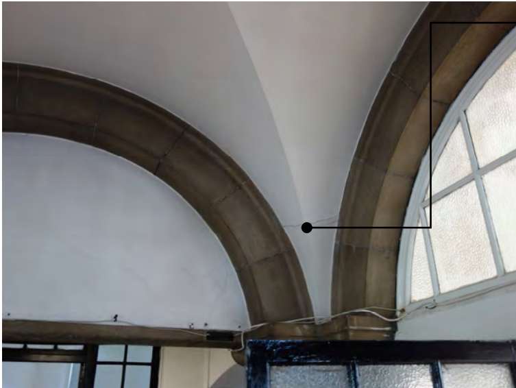
2.8 Cracking in plaster as base of arch.
