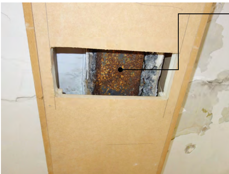
4.10 Light corrosion can be seen to the steelwork over the top of the stair.
