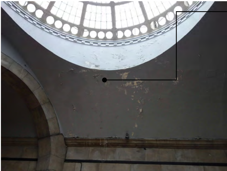
G.5 Water ingress noticeable at high level.
