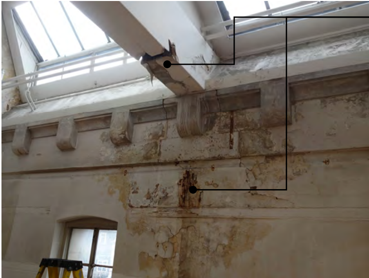
4.2 Corrosion to steelwork and water ingress on the wall is apparent.
