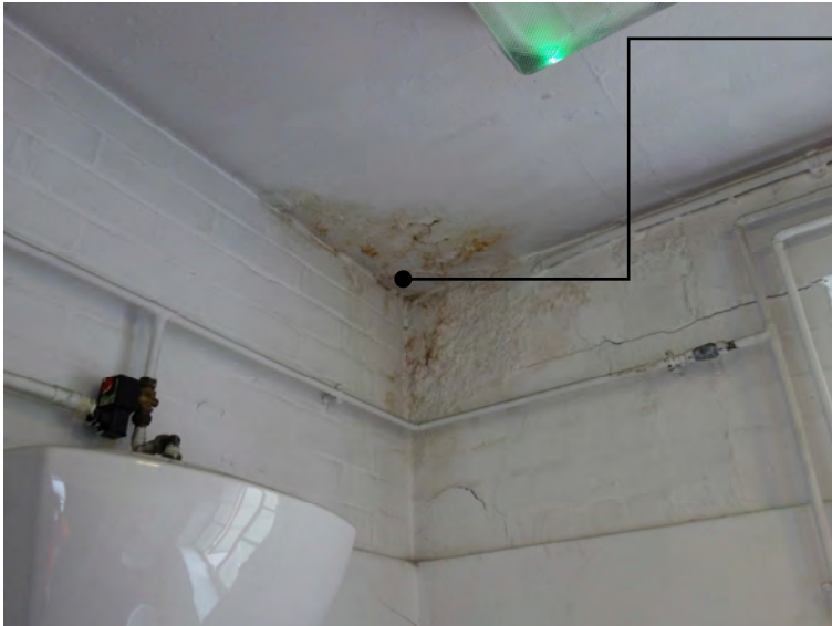
4.8 Water ingress to around slab and wall apparent.
