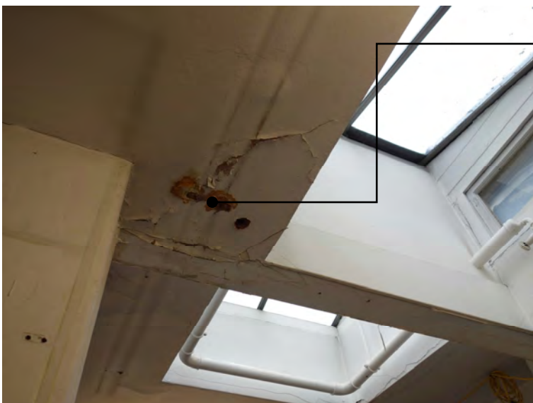
5.5 Rust stains can be seen on the ceiling below an assumed steel joist location.
