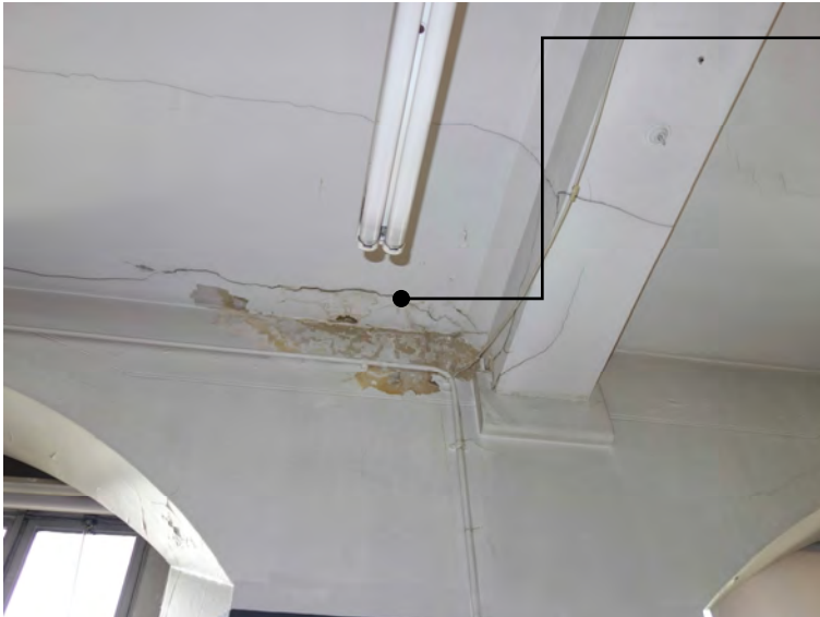
3.4 Cracking along the joist adjacent to the wall can be seen.
