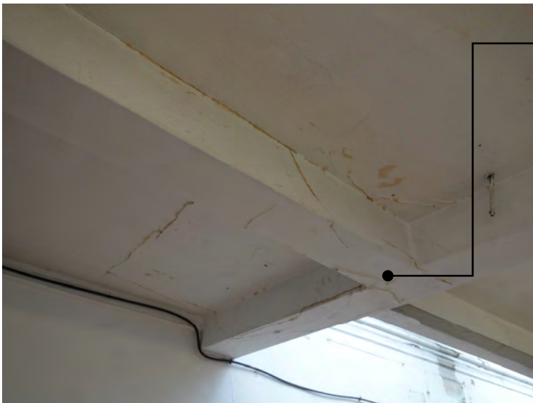
5.9 Water ingress and signs of corrosion apparent on plaster surrounding steel downstand beams.
