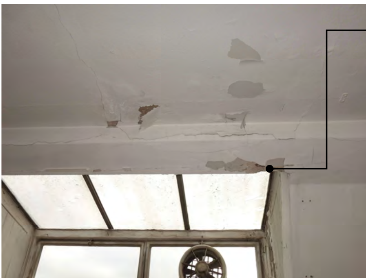
5.12 Cracking can be seen to the bottom of the steel beam running across the roof lights.
