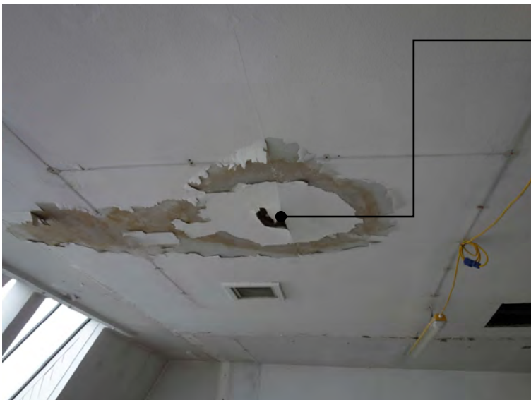
5.15 Water damage and staining to the suspended ceiling suggests water ingress through the structure above.
