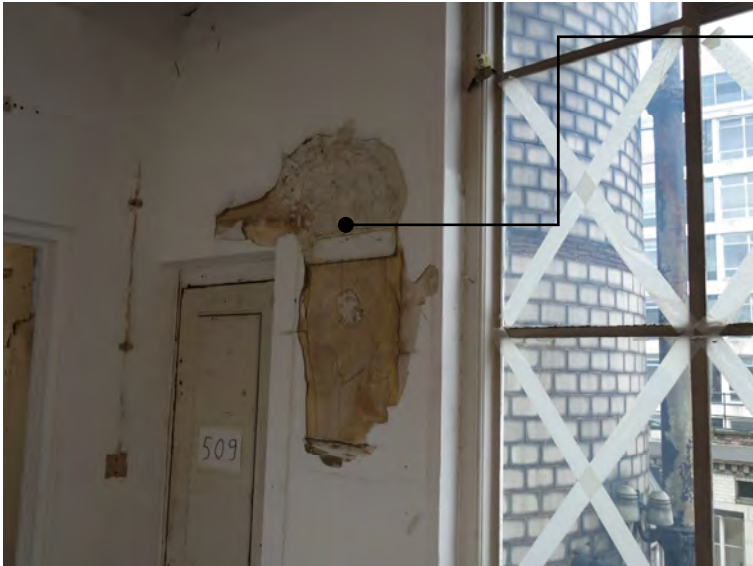
5.3 Plaster swelling seen in wall indicating water ingress.
