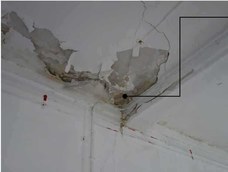
5.13 Plaster swelling and damage seen in slab and adjacent beam indicating water ingress.
