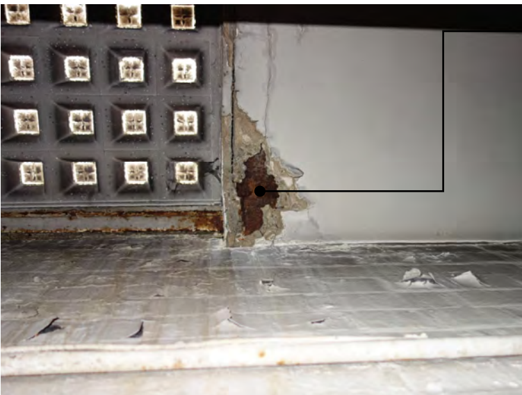
B.3 Corroded steel joist trimming the edge of the pavement light.
