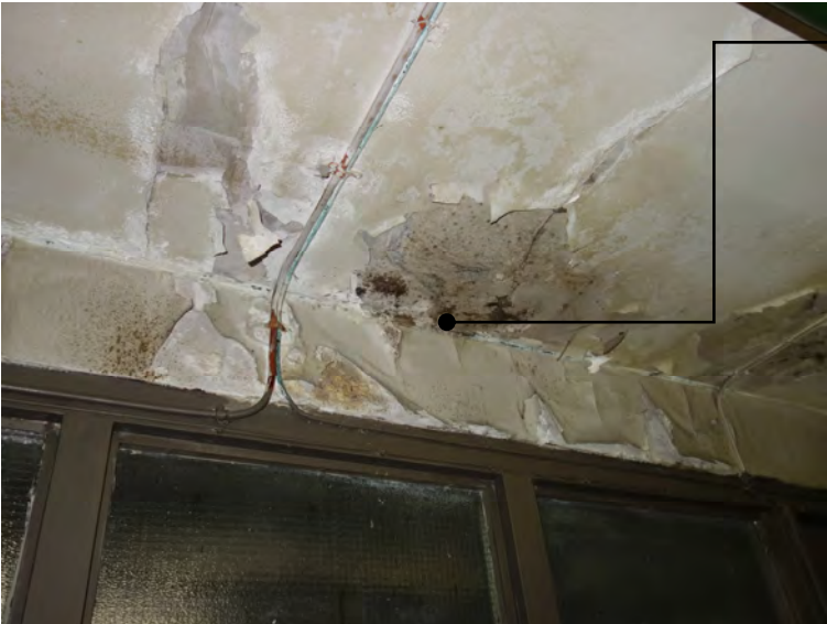
B.2 Significant water ingress is apparent around the beam support.
