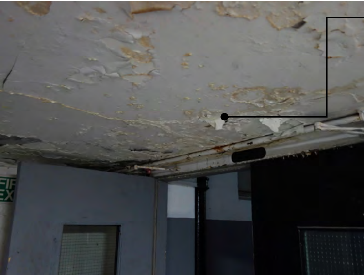
B.8 Water ingress noticeable at high level.
