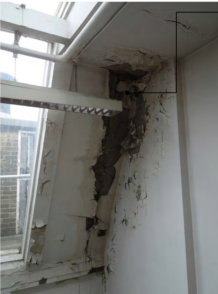
5.17 Water ingress and damage to plaster apparent in mansard and roof slab.
