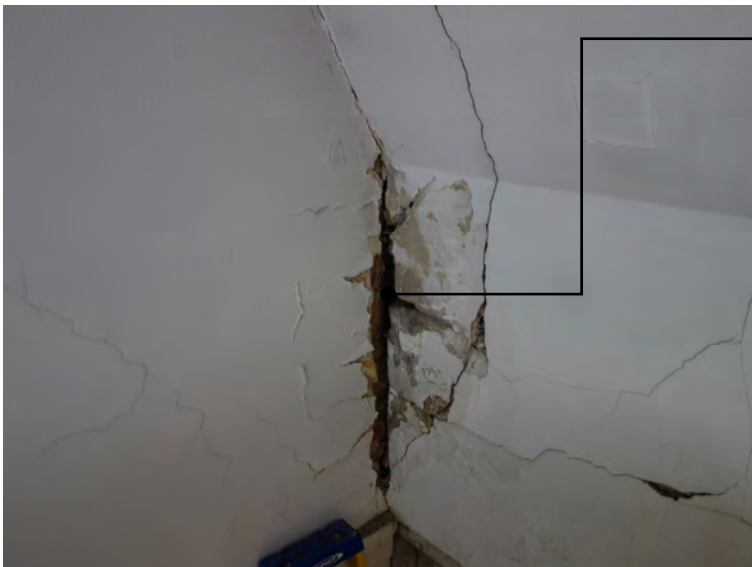
4.4 Damage to the plaster from water ingress is apparent.
