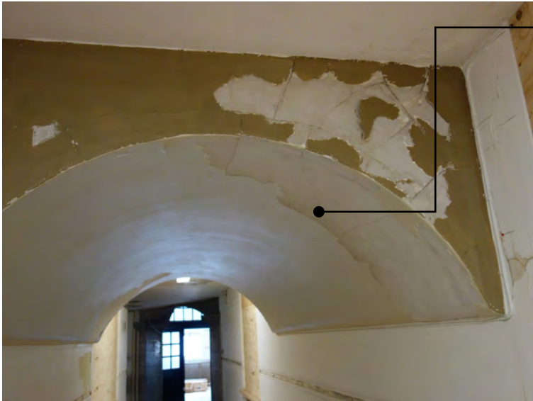
4.13 Cracking is evident on the underside of the arch.
