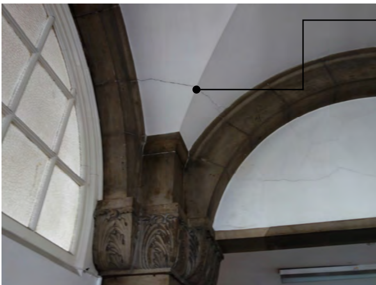
1.1 Cracking in plaster as base of arch.
