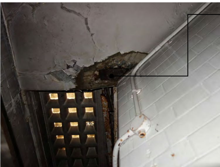
B.4 Corroded steel joist trimming the edge of the pavement light.
