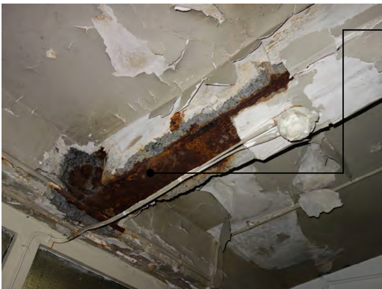
B.2 A beam supporting the underside of the lecture theatre is heavily corroded.
