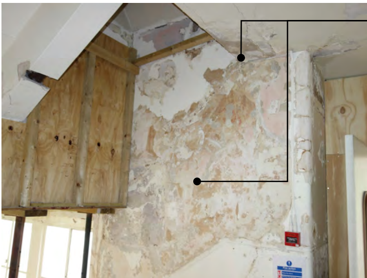
4.14 Heavy water damage apparent to plaster on the wall.
