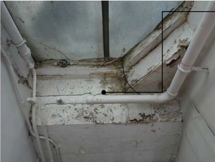
5.18 Water ingress beneath the window is apparent.
