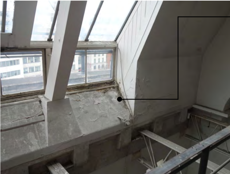
5.16 Swelling and damage to the plaster at the corner of the window suggests water ingress.
