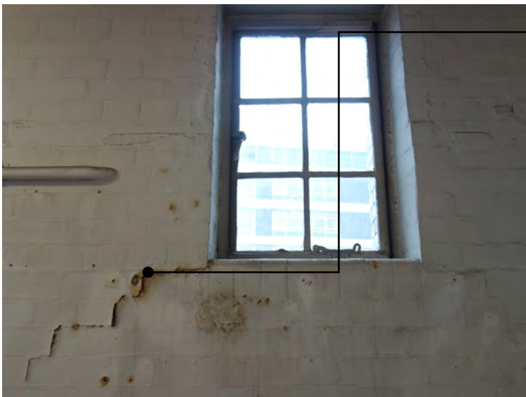
5.4 Large crack to the plaster at the corner of the window.
