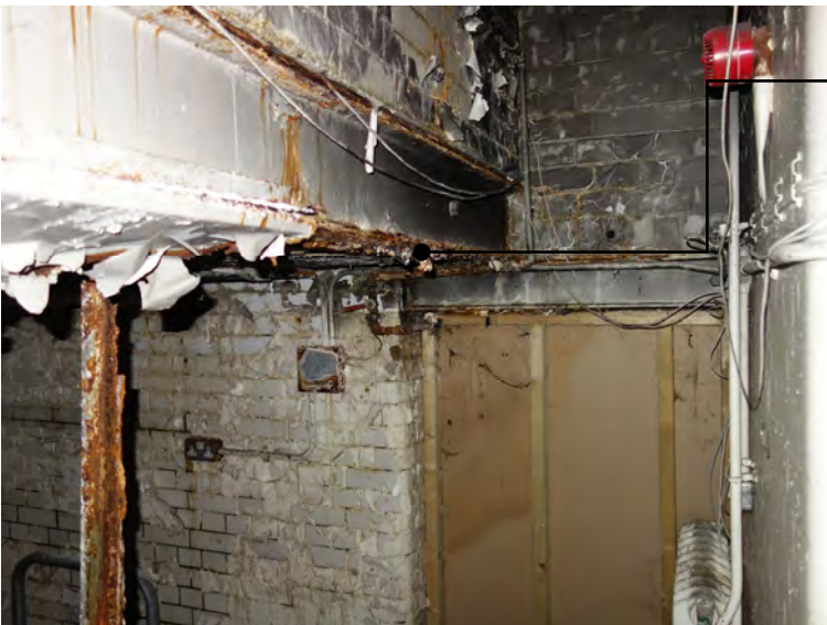
B.10 Water ingress in the vaults had led to significant corrosion and delamination of numerous beams and joists.
