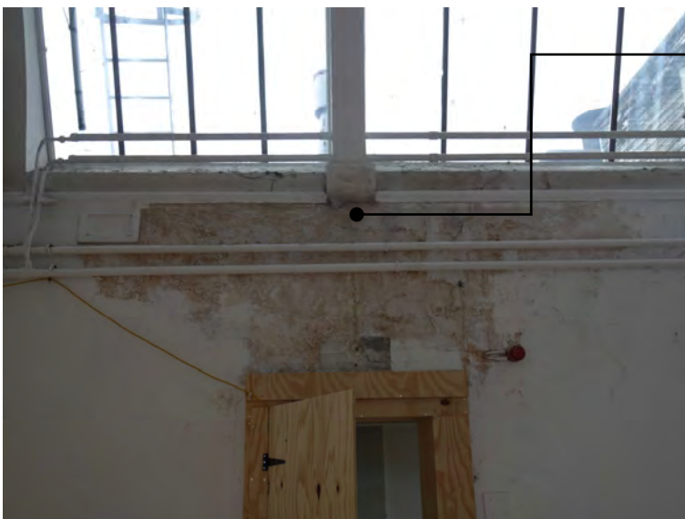
4.12 Damage to the plaster below the high-level windows indicating water ingress.
