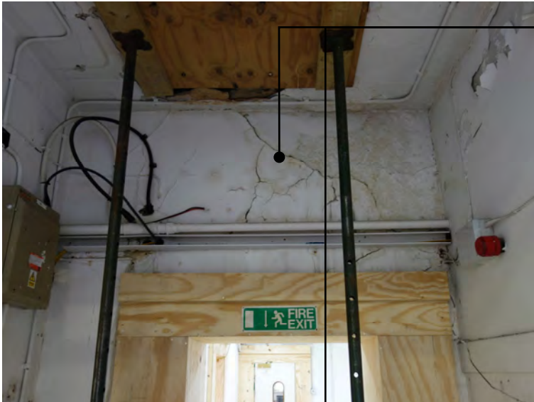
4.11 Significant cracking in plaster due to water ingress apparent.
