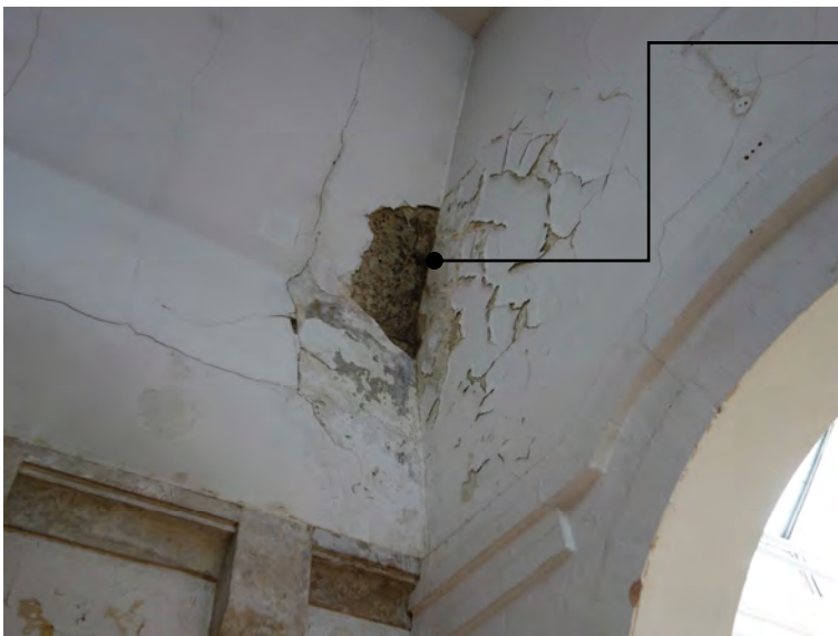
4.3 Damage to the plaster from water ingress is apparent.
