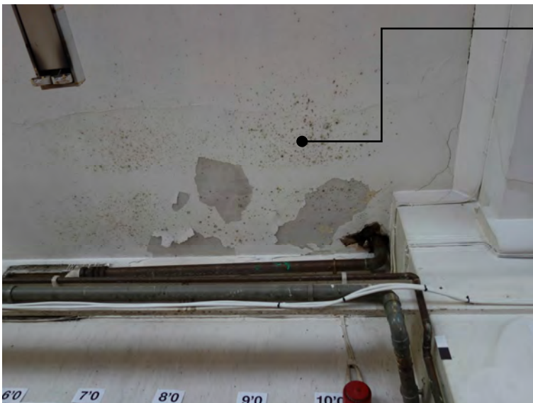
3.5 Mould on the ceiling indicates moisture within the slab.
