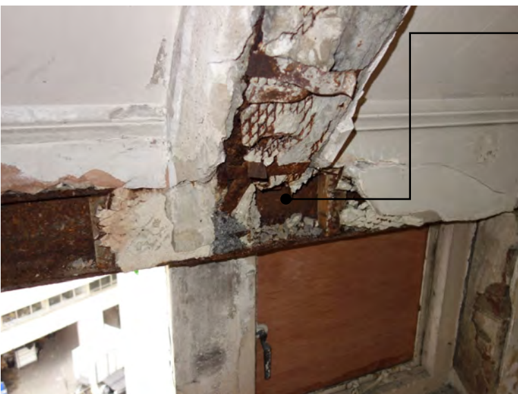
5.20 Heavy corrosion and delamination apparent on steelwork.
