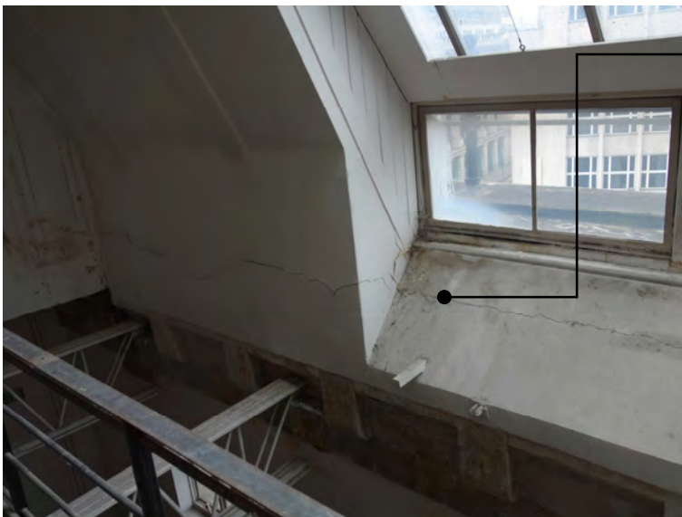
5.14 Cracking along the length of the window and the adjacent section of wall is evident.
