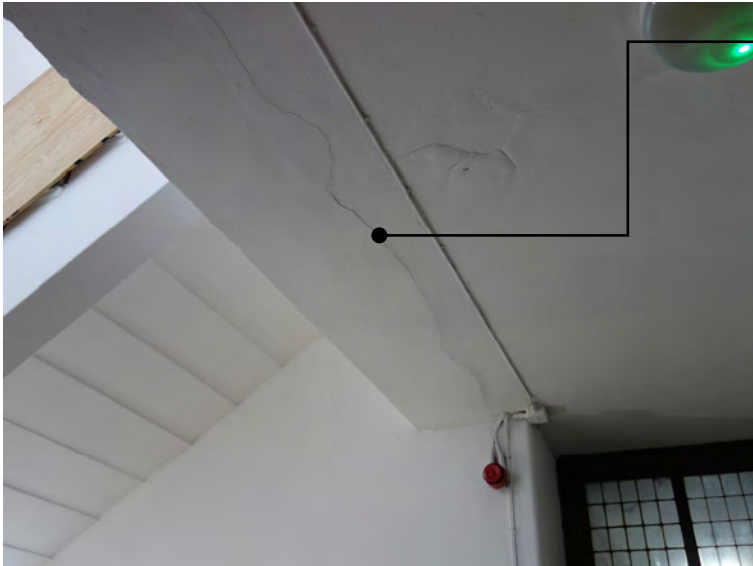
G.2 Cracking is evident to the underside of the beam supporting the stair.
