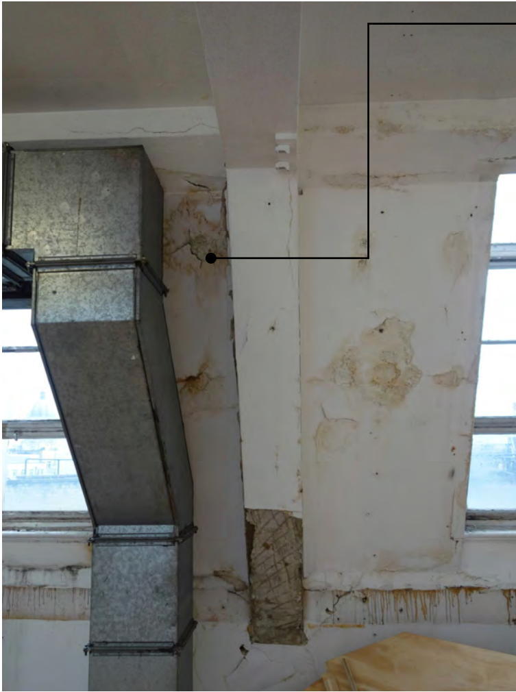
5.8 Plaster swelling seen in wall indicating water ingress.
