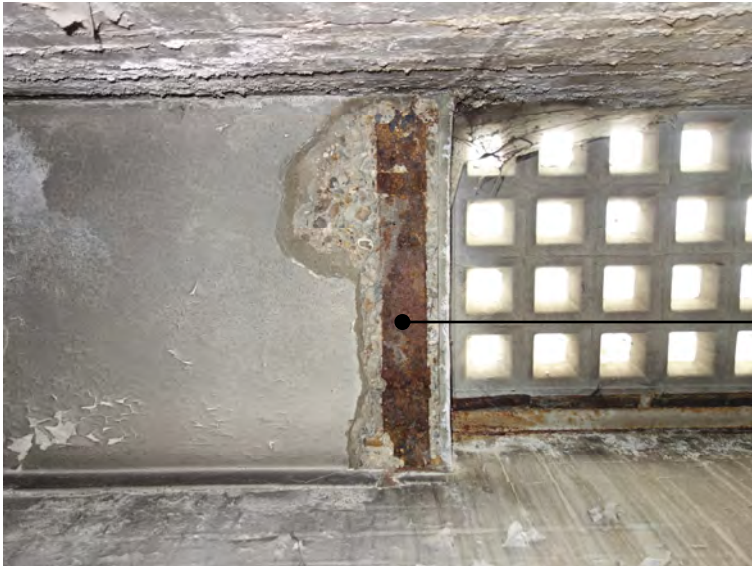
B.1 Corroded steel joist trimming the edge of the pavement light.
