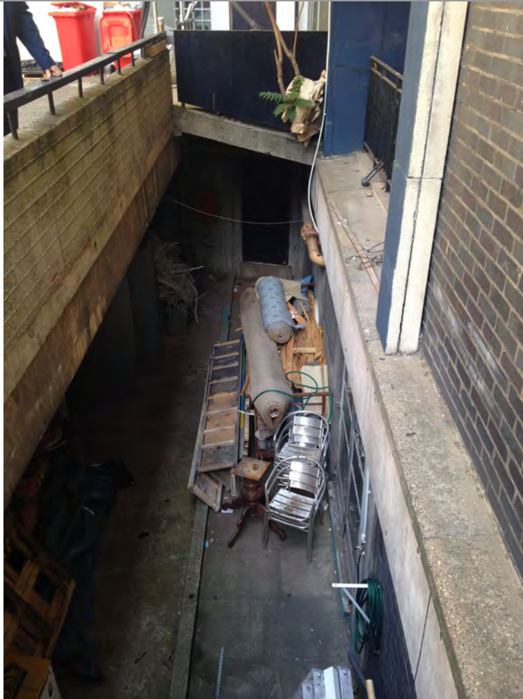
Plate 4 - Foundations of the Red Lion Square building
