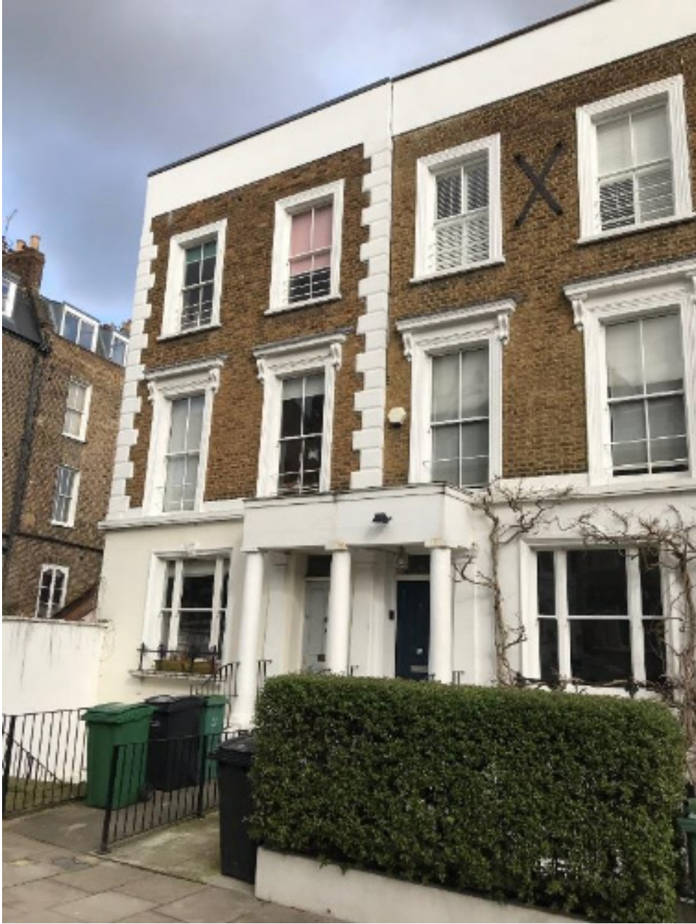
Principal elevation viewed from Berkley Road
